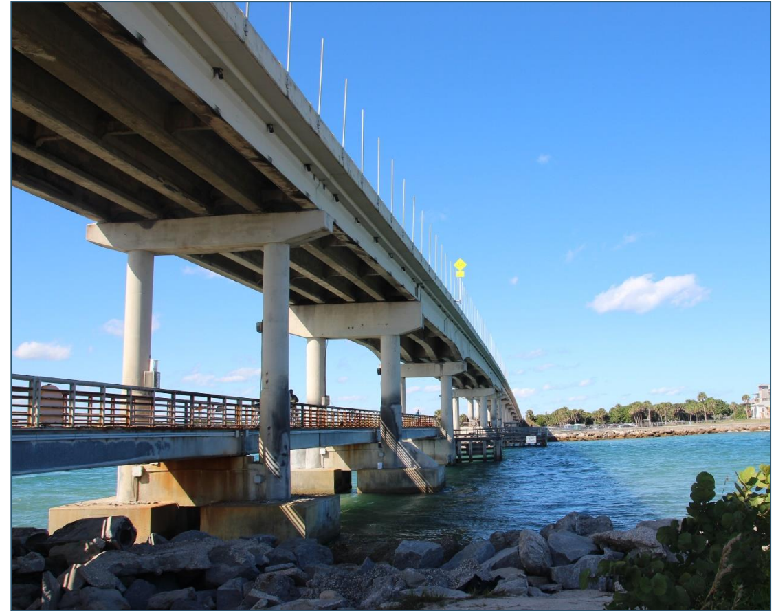
James H. Pruitt Memorial Bridge
