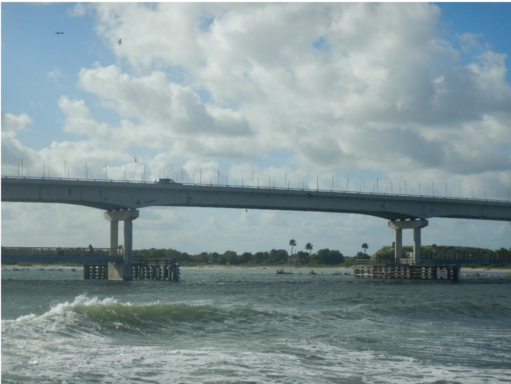
Sebastian Inlet Bridge from the east, facing towards the west.
