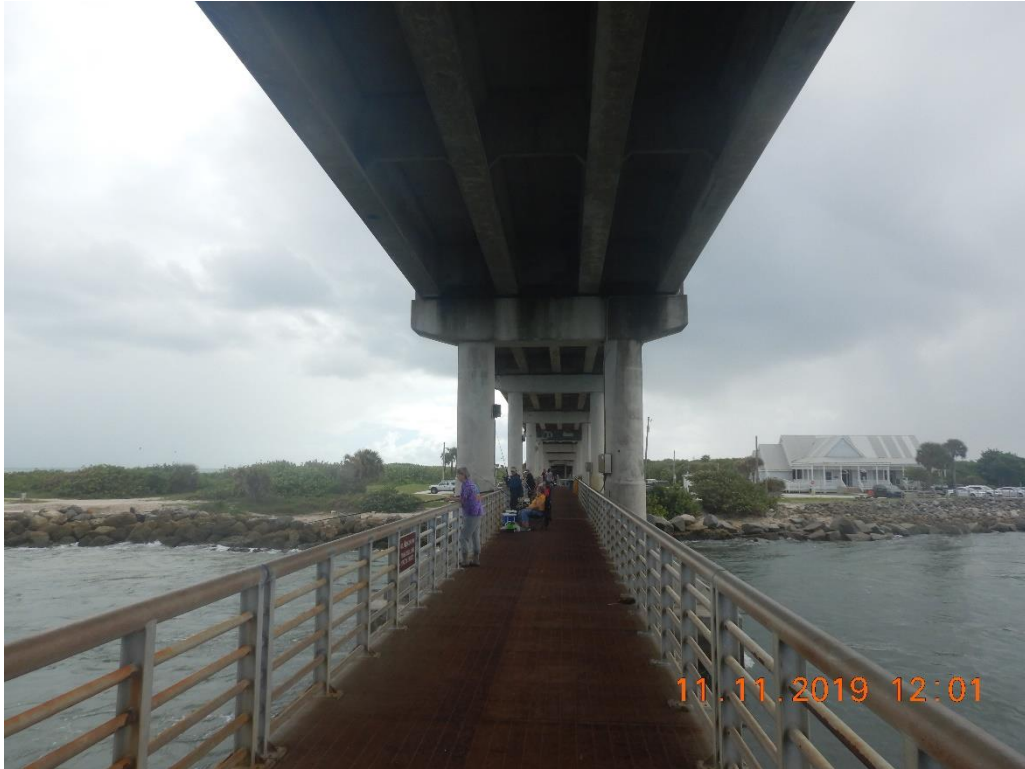
Underdeck of Sebastian Inlet Bridge, facing south along bridge alignment.
