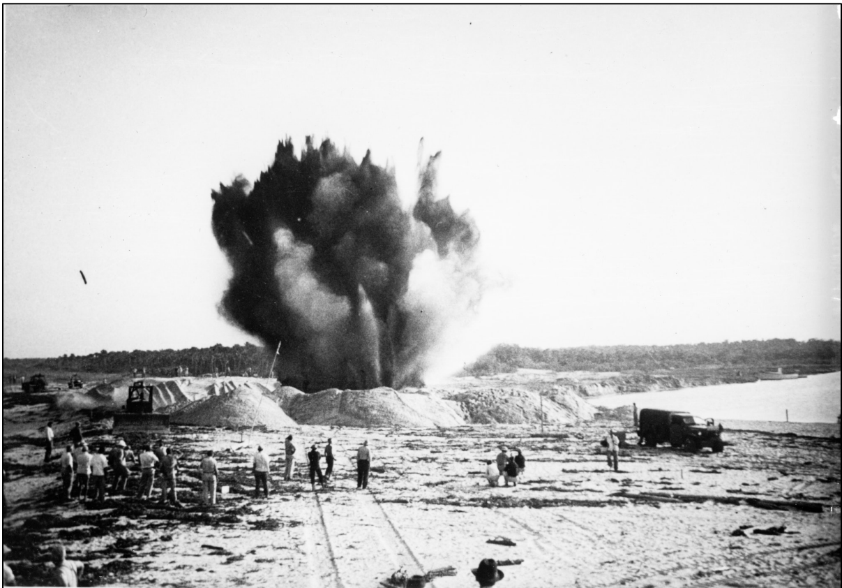
Figure 7: 1947 Photograph Showing Surplus Navy Ordinance Being Utilized to Open the Sebastian Inlet ( Photograph Courtesy of the Sebastian Inlet District )
