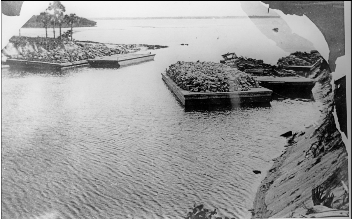
Figure 6: 1923 Photograph showing Barges of Coquina Rock for the 1923 Sebastian Inlet Improvements ( Photo Courtesy of the Sebastian Inlet District )
