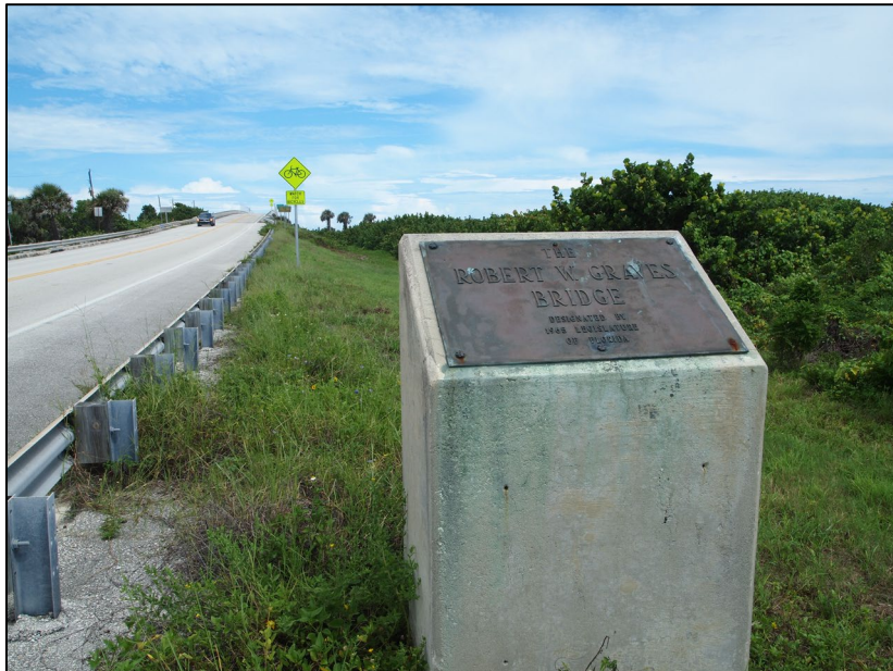
Figure 34: Plaque for the Establishment of the James H. Pruitt Memorial Bridge/FDOT Bridge 880005 (8BR3148/8IR1493), Determined National Register Eligible, facing North
