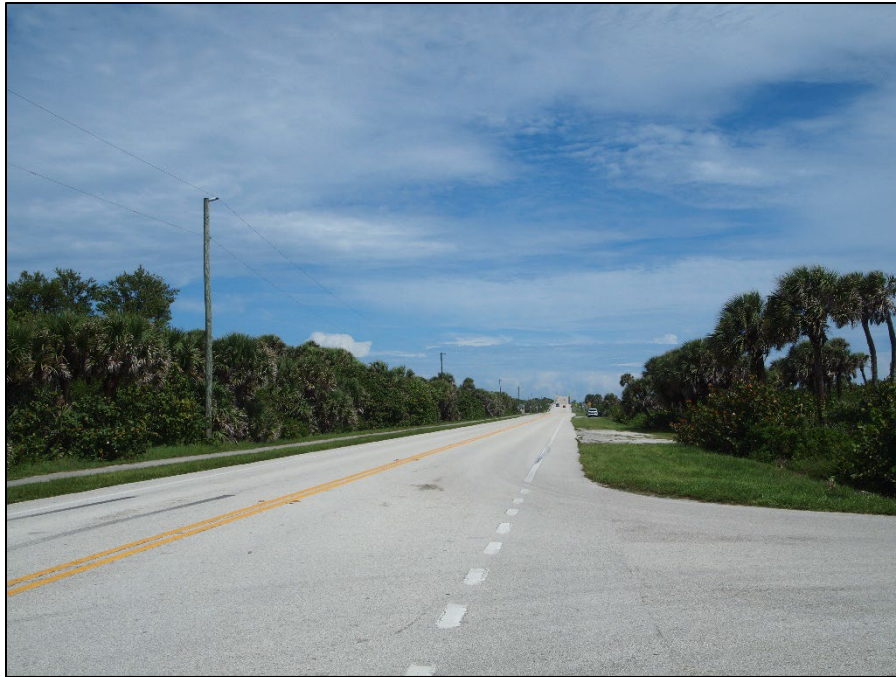
Figure 1: SR A1A (8IR1500), Within the Project APE, Considered National Register Ineligible, facing North
