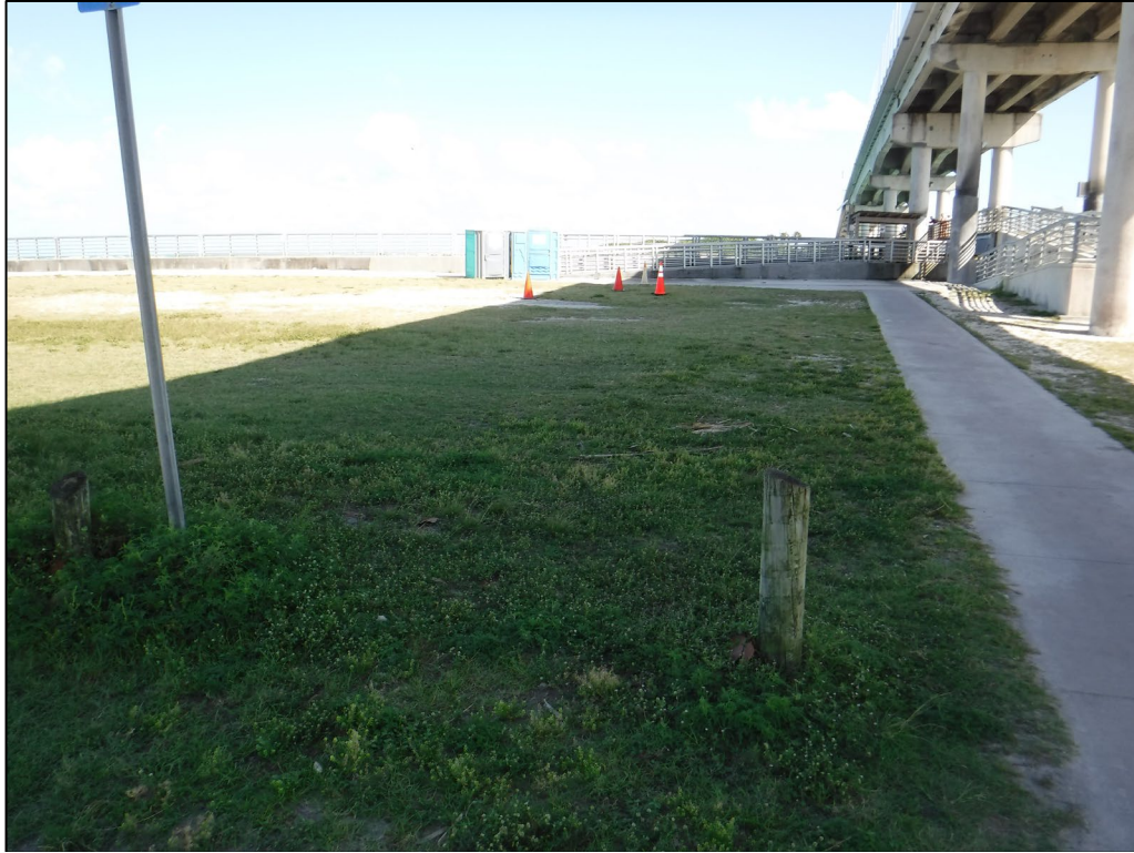
Figure 21: Area Containing Fill Under the Bridge on the North Side of Sebastian Inlet in a Low Probability Zone, Facing South
