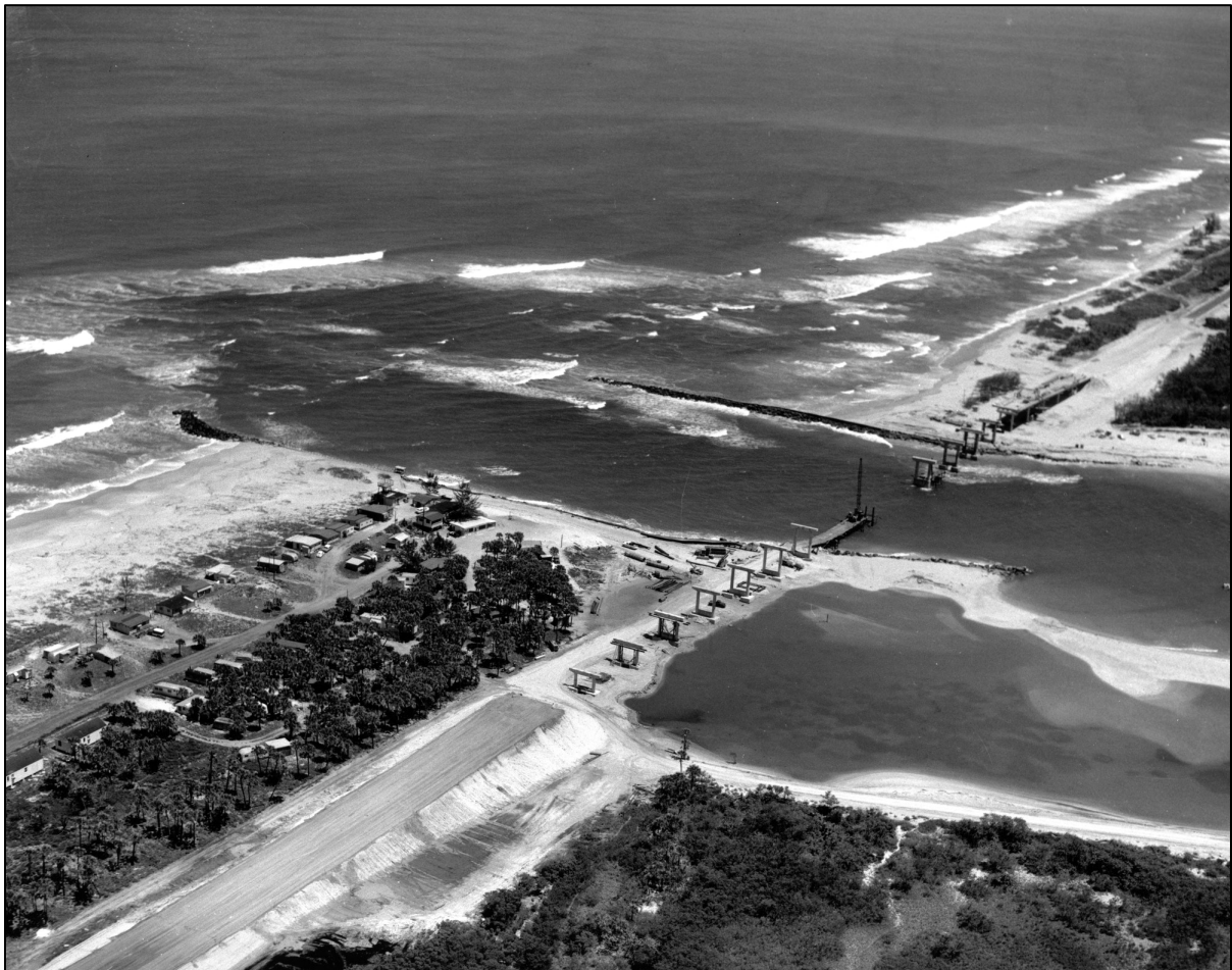
Figure 9: 1964 Aerial Showing the James H. Pruitt Memorial Bridge (FDOT Bridge No. 880005) Under Construction, facing southeast ( Aerial Courtesy of the Sebastian Inlet District ).
