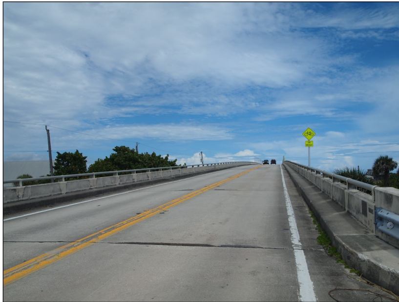
Figure 32: The Southern Portion (Indian River County) of the James H. Pruitt Memorial Bridge/FDOT Bridge 880005 (8IR1493), Determined National Register eligible, facing North
