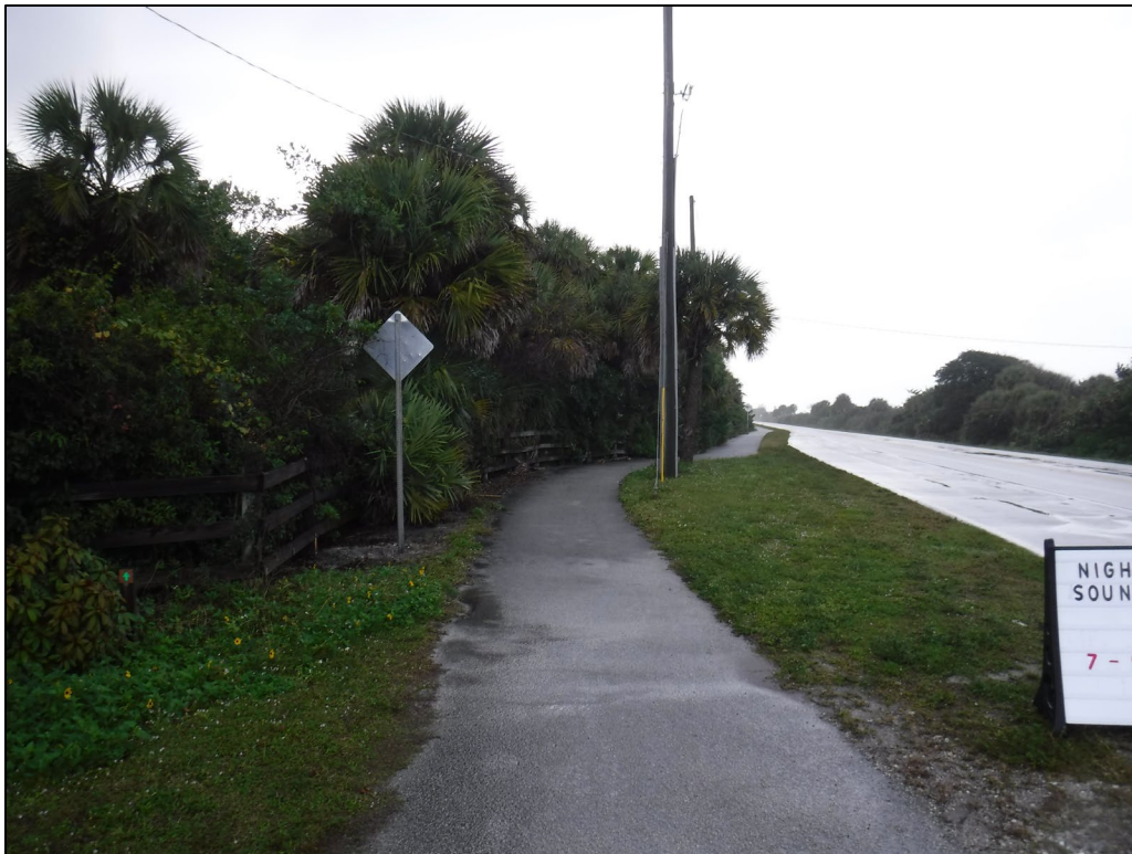
Figure 18: Sidewalk in High Probability Zone North of Brevard County Entrance to the Sebastian Inlet State Park on the West Side of SR A1A, Facing North-Northwest
