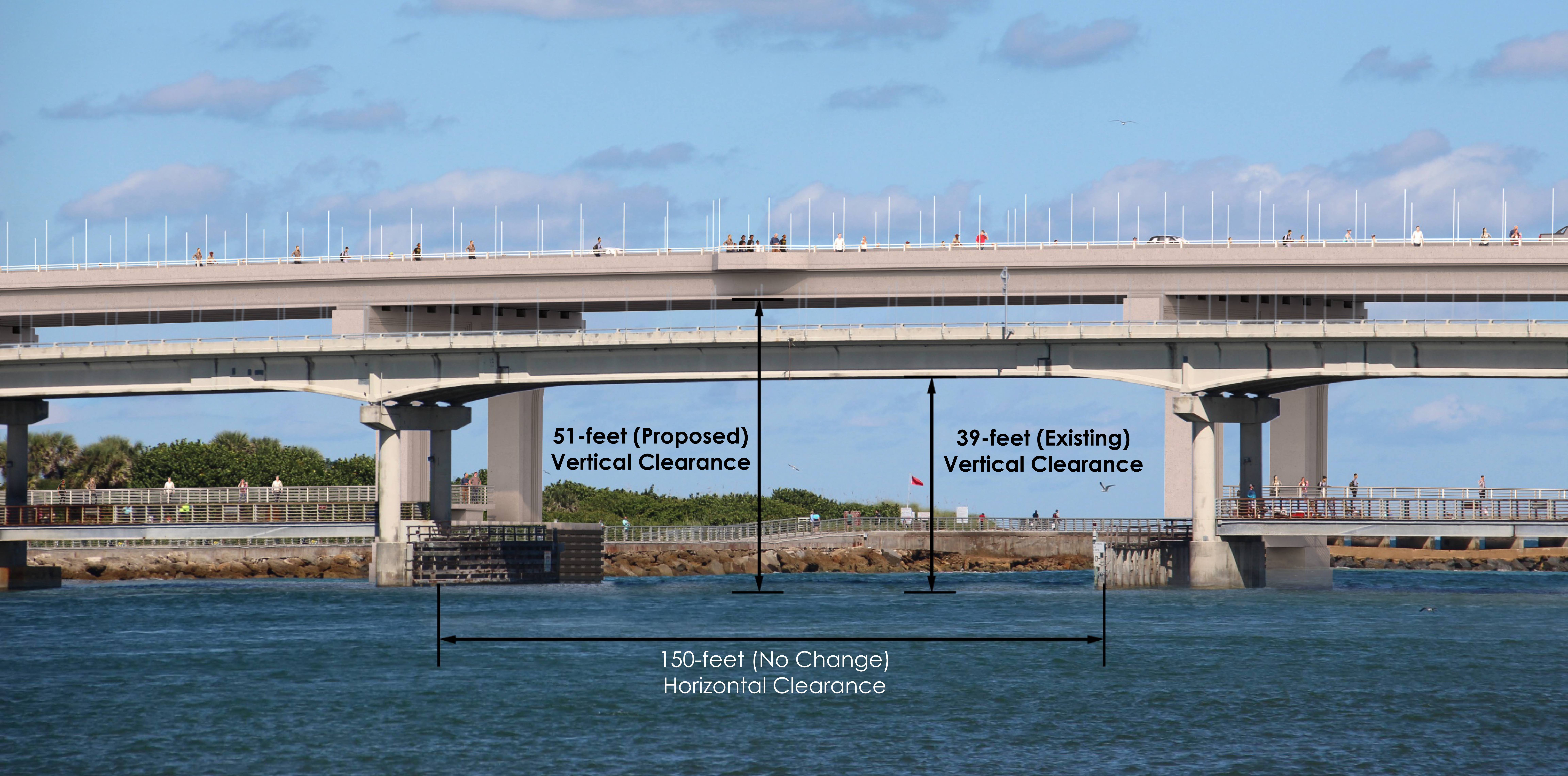
Looking Northeast from Southwest Side of Inlet
