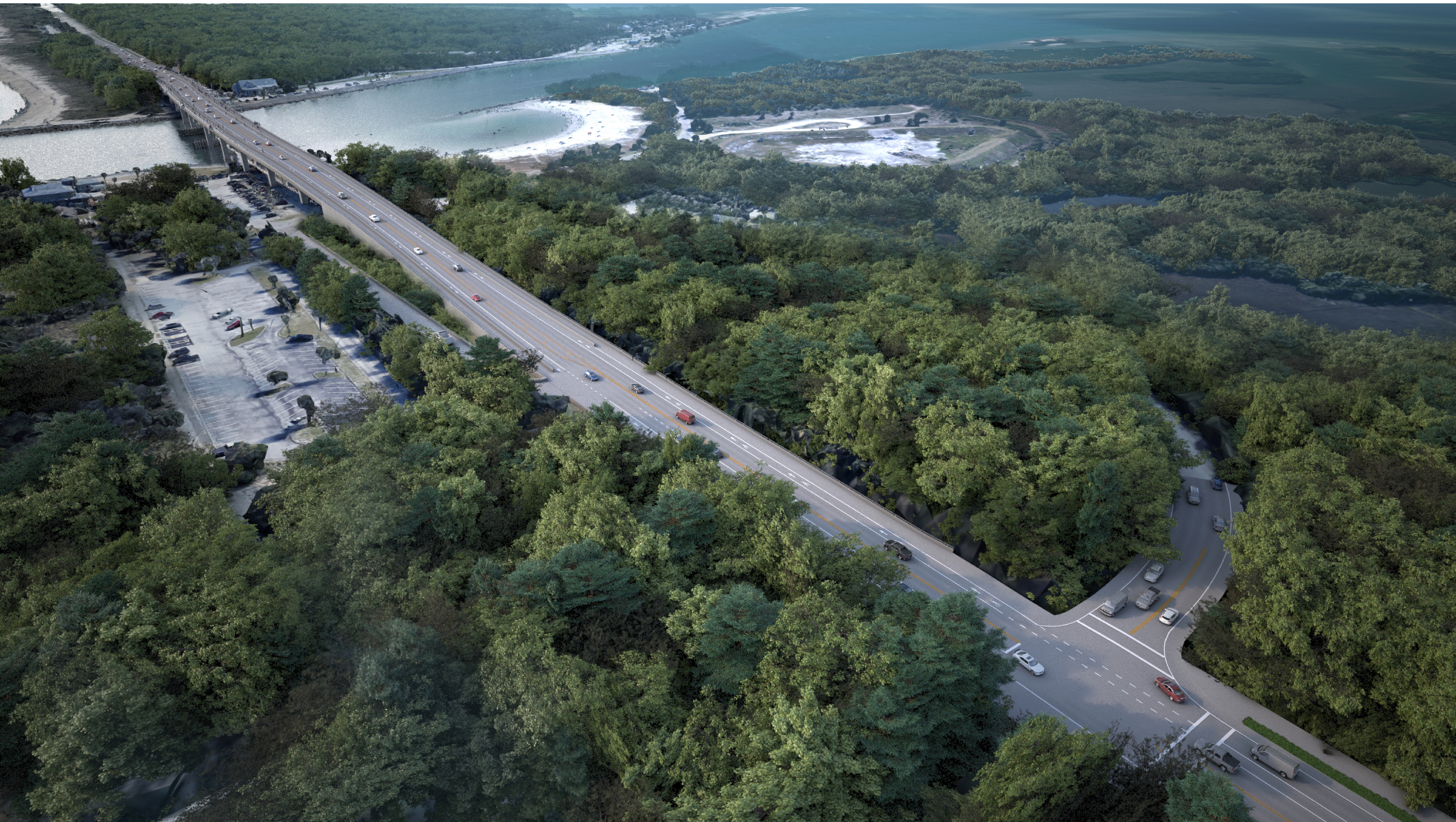
Looking South from North Park Entrance
