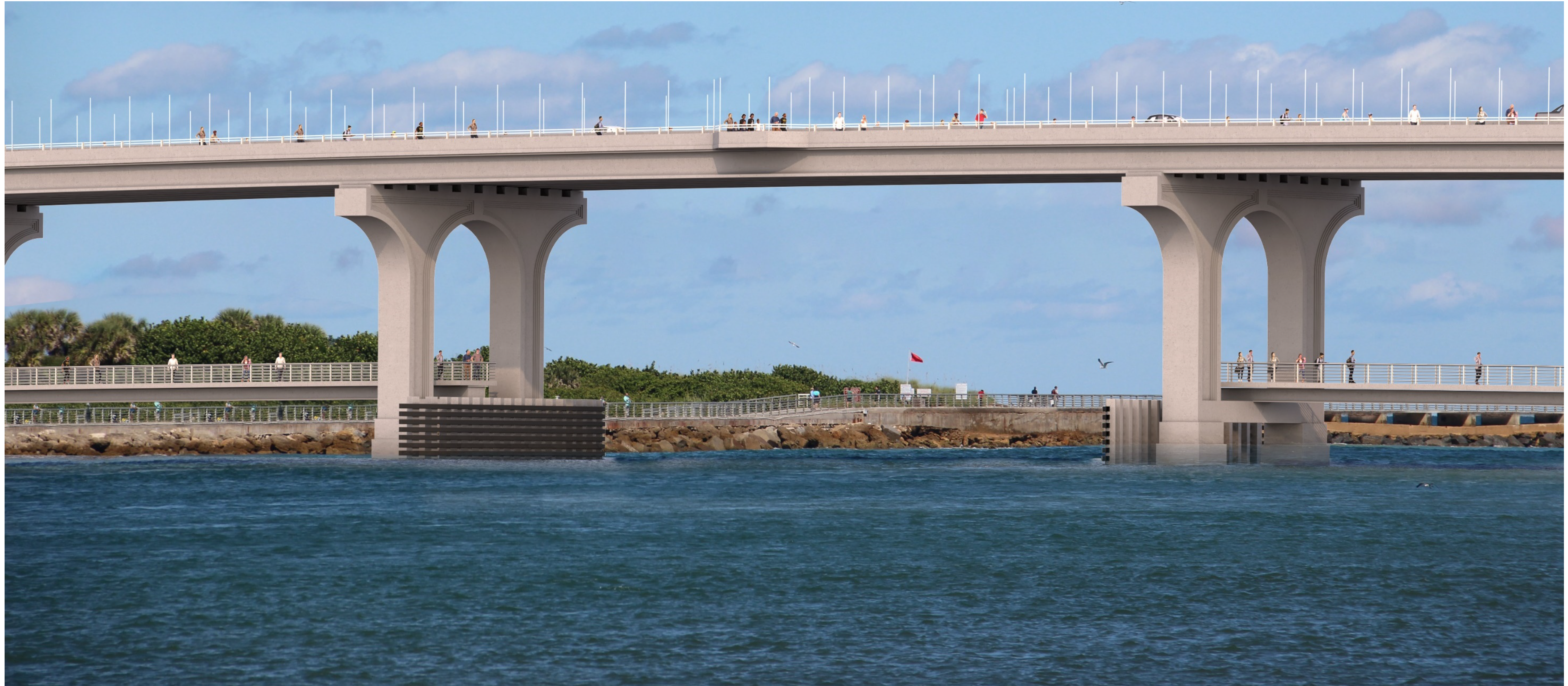
View Looking Northeast from Southwest Side of Inlet
