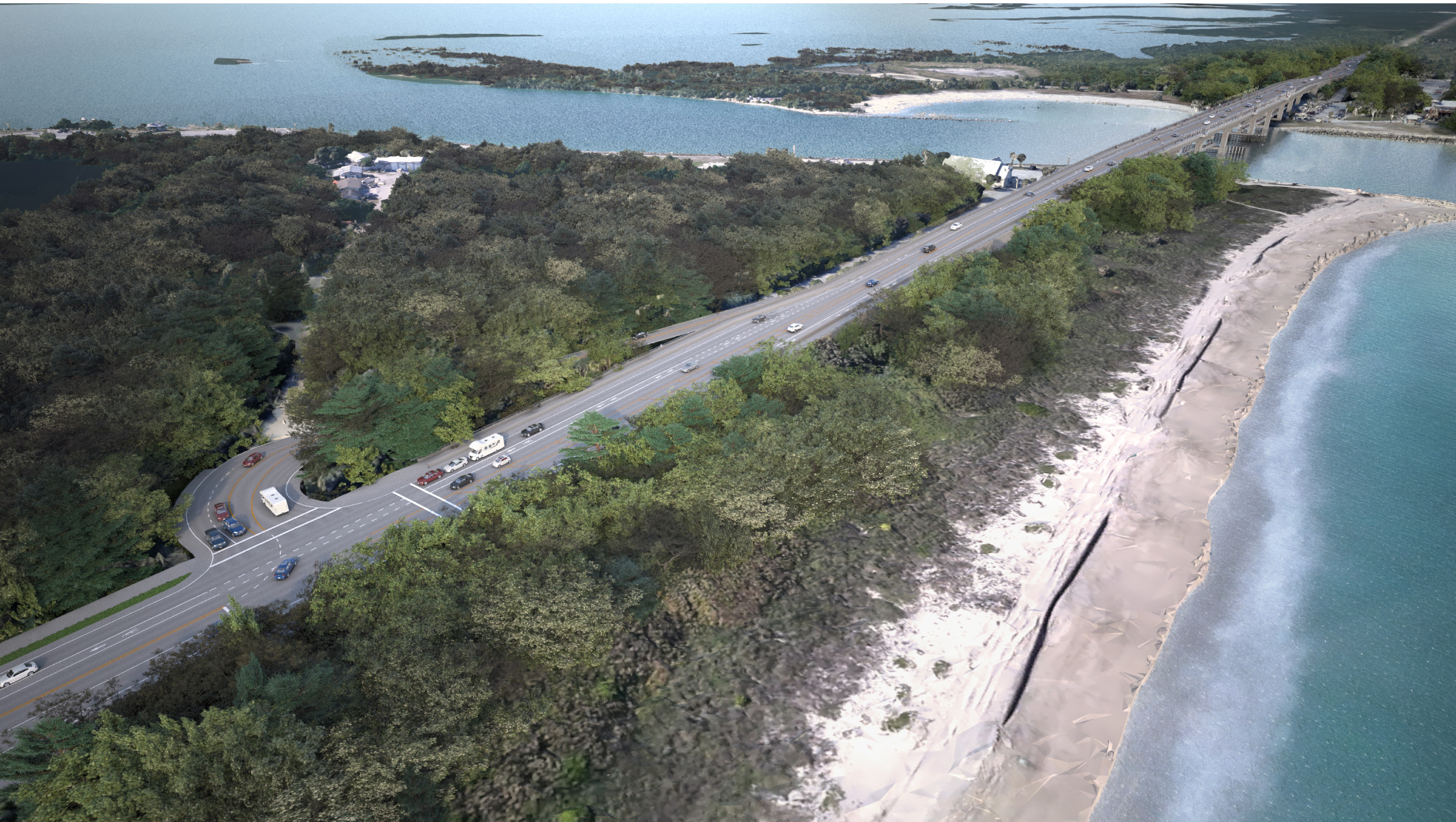
Looking North from South Park Entrance
