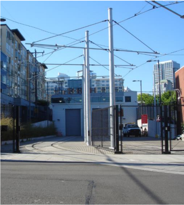
MOF Entrance from Street
