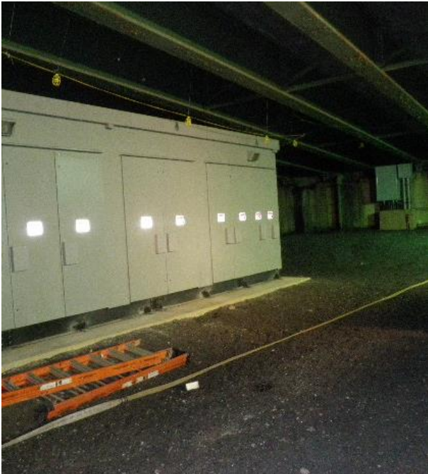
TPSS Beneath Bridge
