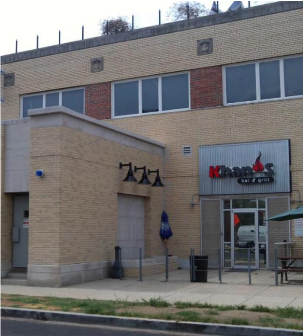
TPSS Integrated within Public Space
