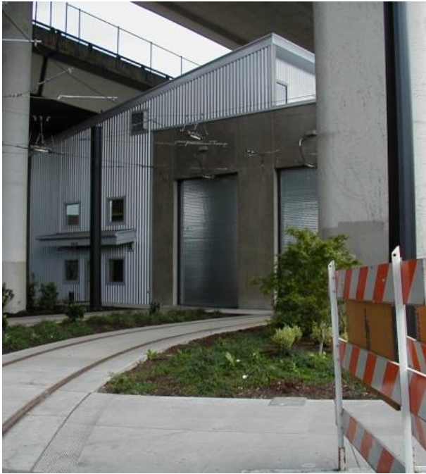
MOF Beneath Interstate
