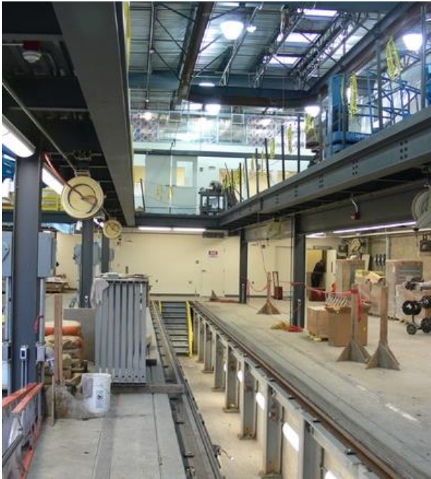
Narrow Maintenance Pit
