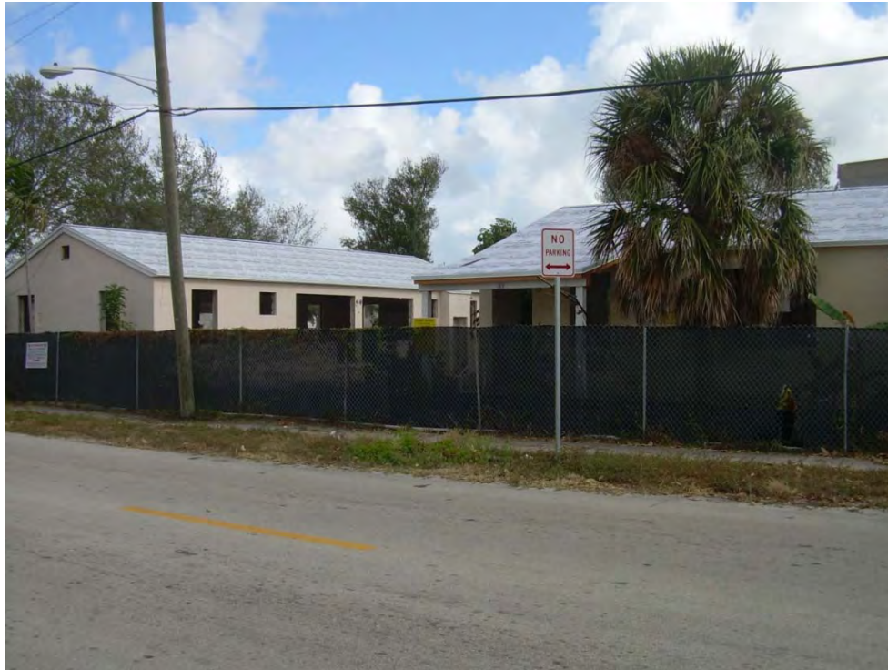
Formerly National Register-listed and currently only three buildings remain after demolition.
