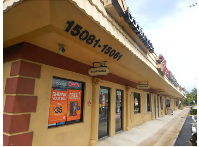
8PB19604_b Facing Northwest
