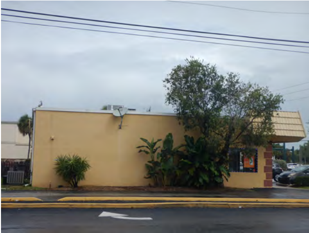
8PB19604_c Facing North
