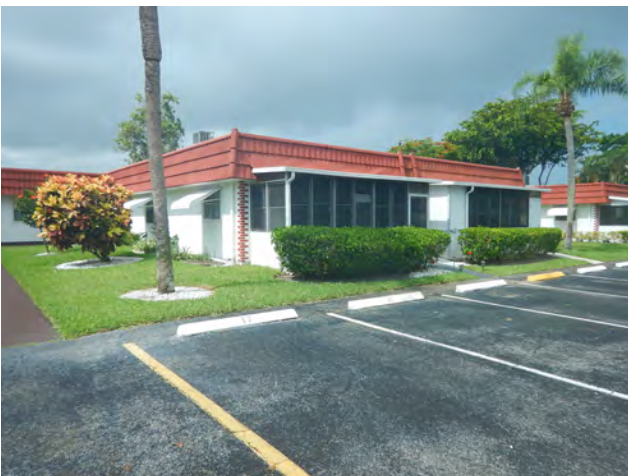
8PB20180_e Facing Southwest
