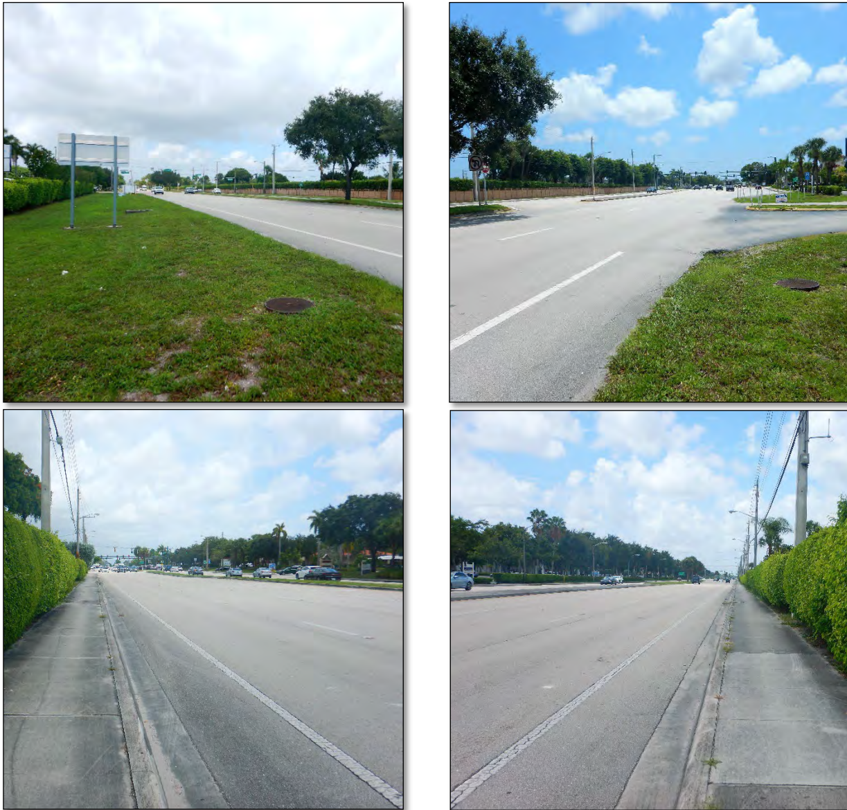
Figure 9. Representative views of the Atlantic Avenue PD&E APE. Atlantic Ave facing west (top left) and east (top right). S. Jog Road facing south (bottom left) and north (bottom right).
