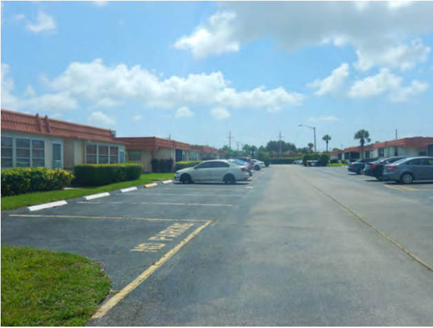
8PB20180_a Facing East
