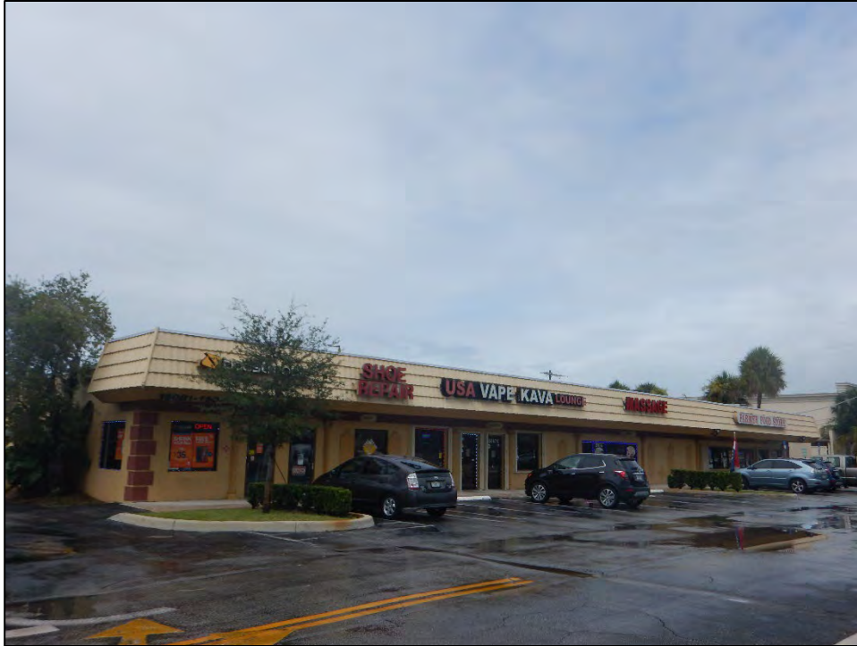
Figure 11. Resource 8PB19604, facing northwest.
