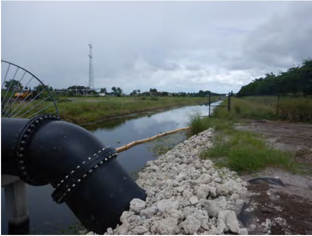
8PB07707_a Facing Northwest
