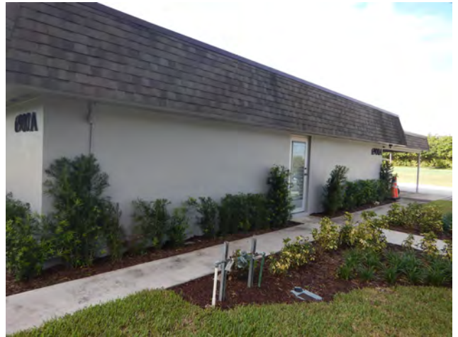
8PB20177_b Facing Southwest
