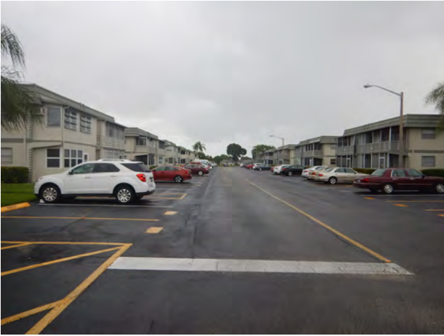
8PB20180_g Facing North
