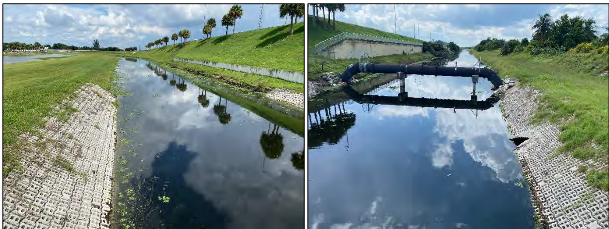
Figure 13. Resource 8SE07704 as seen from SR 806/Atlantic Avenue within the APE, facing north (left) and facing south (right).
