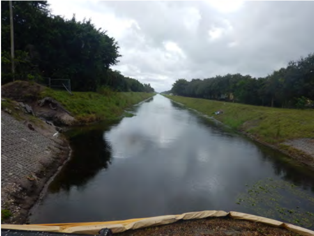
8PB07707_c Facing South
