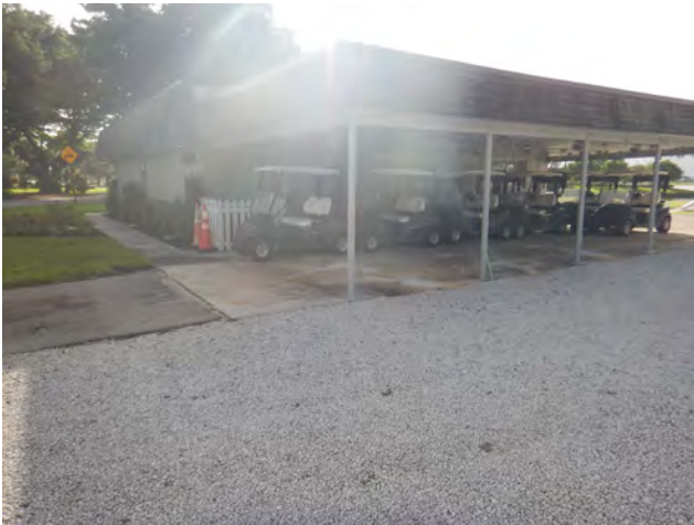
8PB20177_c Facing East
