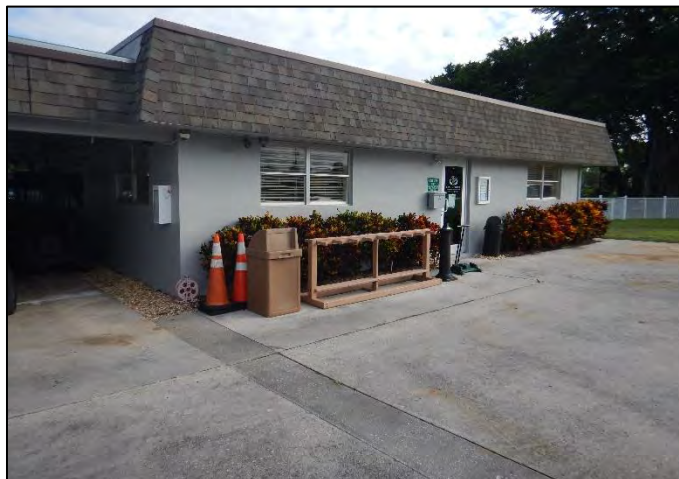
Figure 11. Resource 8PB20177, an example of Masonry Vernacular, view facing northeast.
