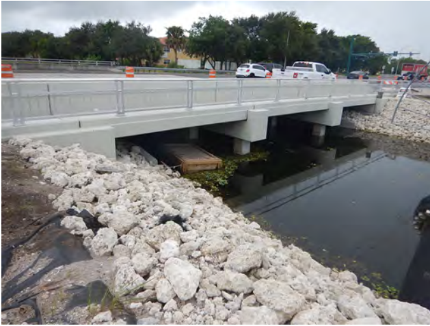
8PB20174_a Facing Southwest
