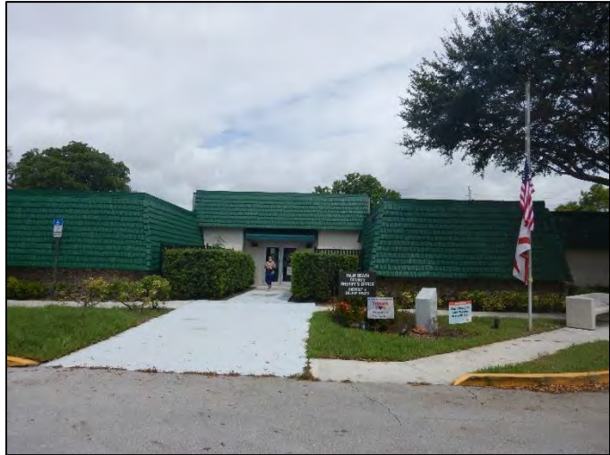
Figure 12. Resource 8PB20175, an example of the Neo-eclectic style, view facing north.
