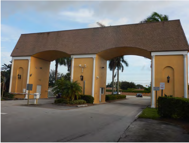
8PB20180_a Facing North
