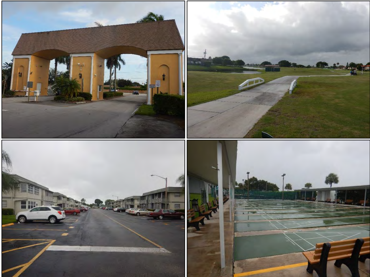
Figure 17. Representative views of Resource Group 8PB20180. Top left, main entry, facing north; top right, par-3 golf course, facing south; bottom left, condominiums along Monaco Court, facing north; bottom right, shuffleboard court, facing east.
