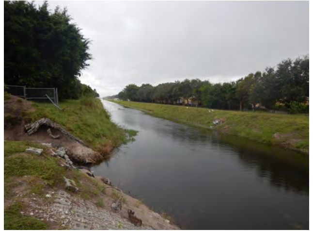
8PB07707_b Facing Southwest
