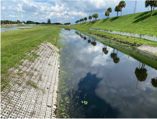
8PB07704_a Facing North
