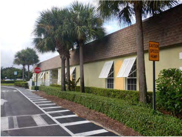
8PB20178_a Facing Southwest
