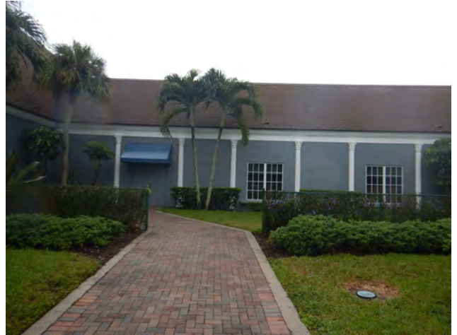
8PB20179_d Facing South
