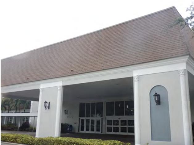
8PB20179_e Facing Southeast
