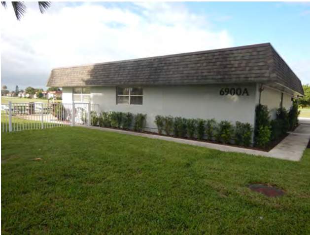
8PB20177_a Facing West
