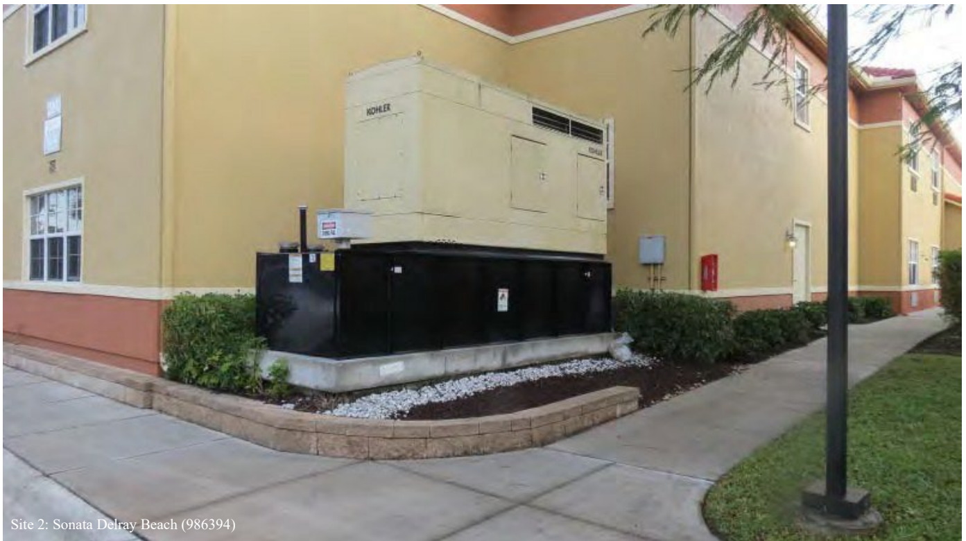
Photo 2: Facing NW from parking area at Sonata Delray Assisted Living Facility. Located south of project corridor. Tank is an attached AST beneath the generator. Below generator tank is larger than usual. Likely the one registered tank. Well Maintained, no evidence of discharge. No expected project impact.
