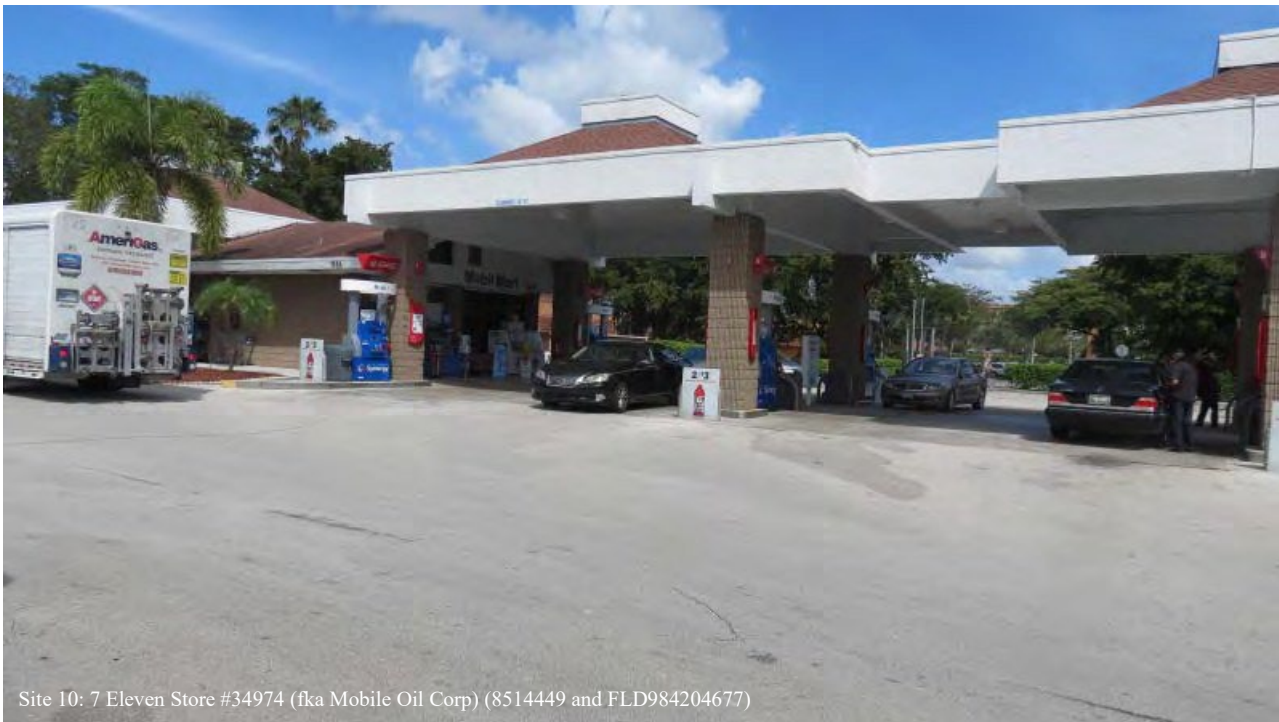
Photo 14. Facing NNW from near West Atlantic Avenue ROW. Site 10 tanks are beyond fuel pumps on back of property. Tanks are approximately 166 feet north of project ROW. Low potential to impact project.
