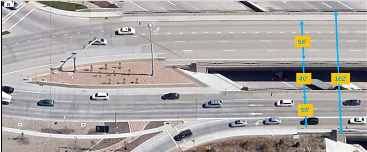
Exhibit 7-13. Cross-sectional distances for a shifted alignment with no reverse curves between crossovers (Pioneer Crossing, American Fork, UT). (26)
