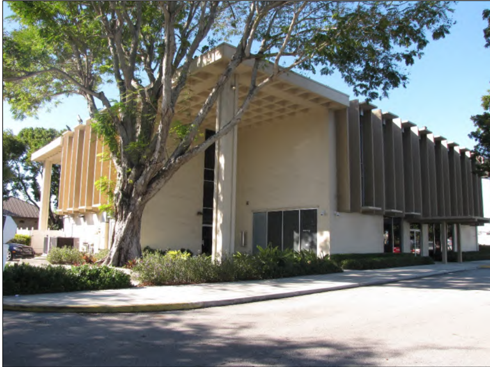
Figure 5: Entry under coffered flat roof extension on southeast corner of First Federal Savings and Loan Association (8PB18601), facing Northwest.
