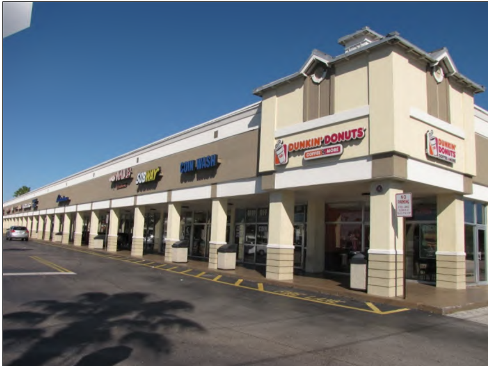
Figure 10-24 Lantana Shopping Center (8PB18605), c. 1960, facing Northeast
