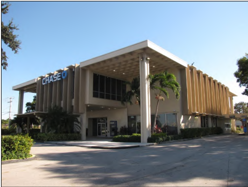
Figure 1: First Federal Savings and Loan Association (8PB18601), c. 1964, is considered eligible for listing in the National Register, facing Southeast
