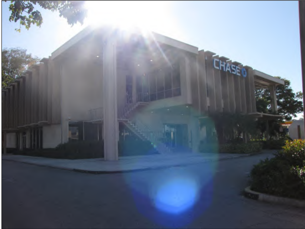
Figure 6: Northeast corner of First Federal Savings and Loan Association (8PB18601), second story entry and open exterior staircase, facing Southwest
