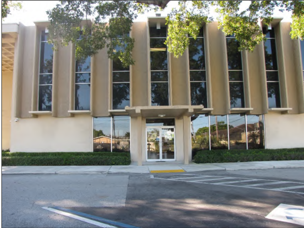
Figure 4: Boxed windows and concrete entry canopy on east façade of First Federal Savings and Loan Association (8PB18601), facing West
