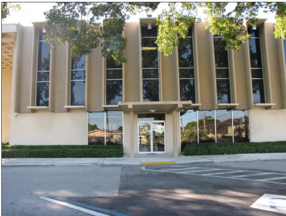
Figure 10-9 Boxed windows and concrete entry canopy on east façade of First Federal Savings and Loan Association (8PB18601), facing West
