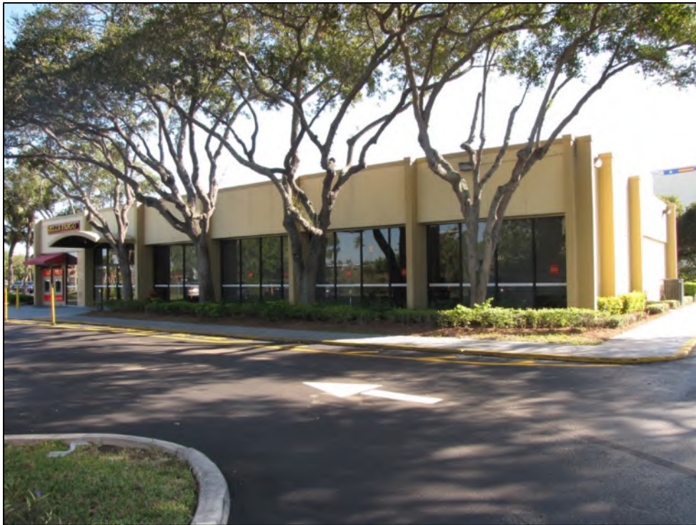
Figure 10-20 1500 W Lantana Road (8PB18600), c. 1963, facing Southeast
