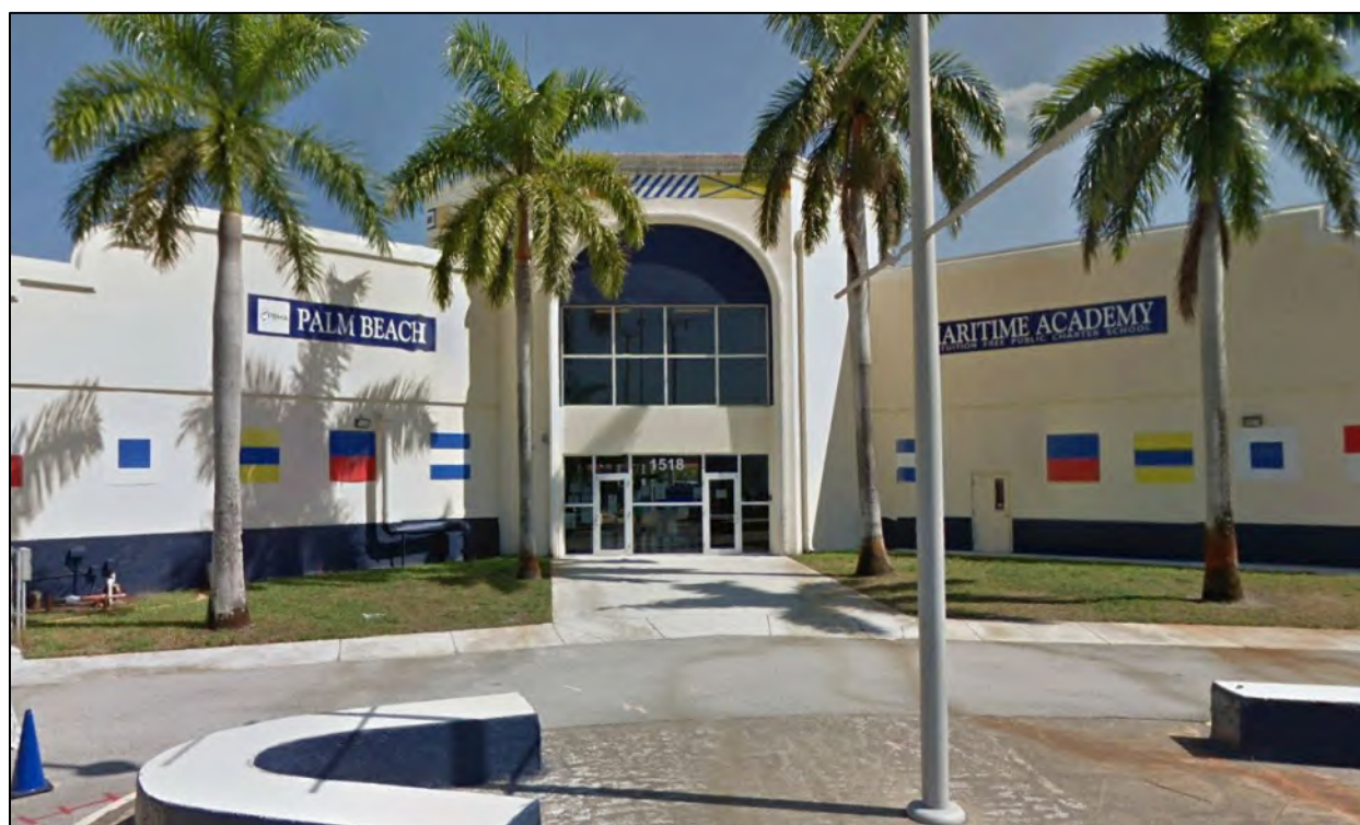
Site # 7 – Former Location of dry cleaners
