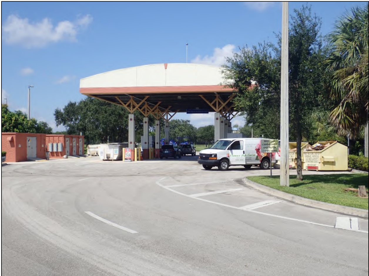
Site # 8 – Solid Waste Authority of PBC-Central County Transfer Station
