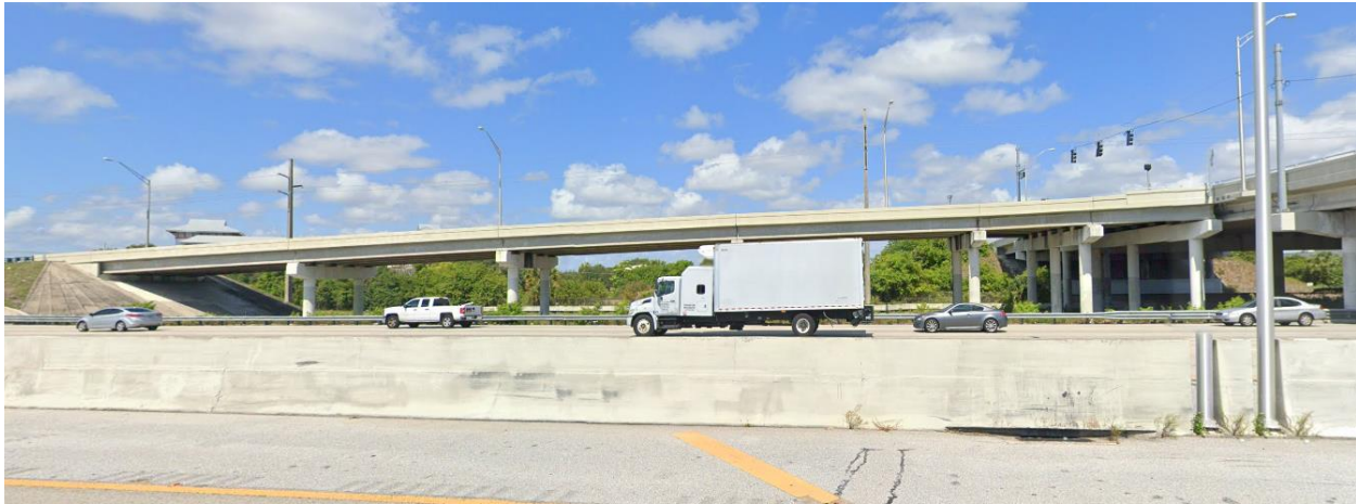
Figure 5-2 Existing Conditions - SR 9/I-95 SB On-Ramp Bridge (930275)
