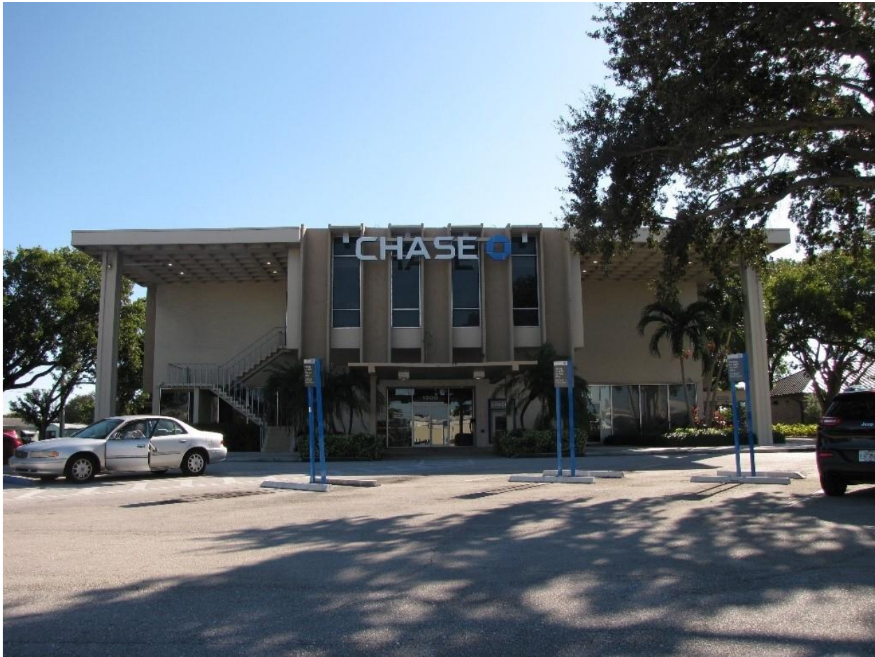
Figure 5 Existing Conditions - First Federal Savings and Loan Association
