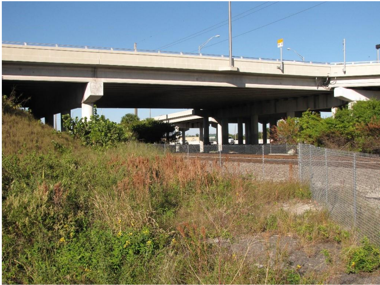
Figure 2 Existing Condition - Seaboard Air Line Railroad
