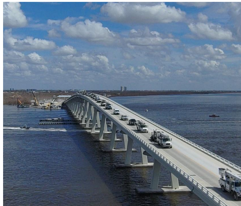
SASHTO Quality of Life/Community Development Award for Sanibel Island Emergency Access
