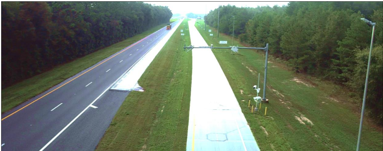
Figure 7. Ramp WIM with size verification devices mounted on overhead structure.
