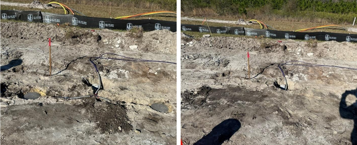
Figure 9 Installation of Earth Pressure Cell
