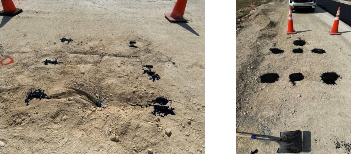
Figure 10 Installation of Asphalt Strain Gauge
