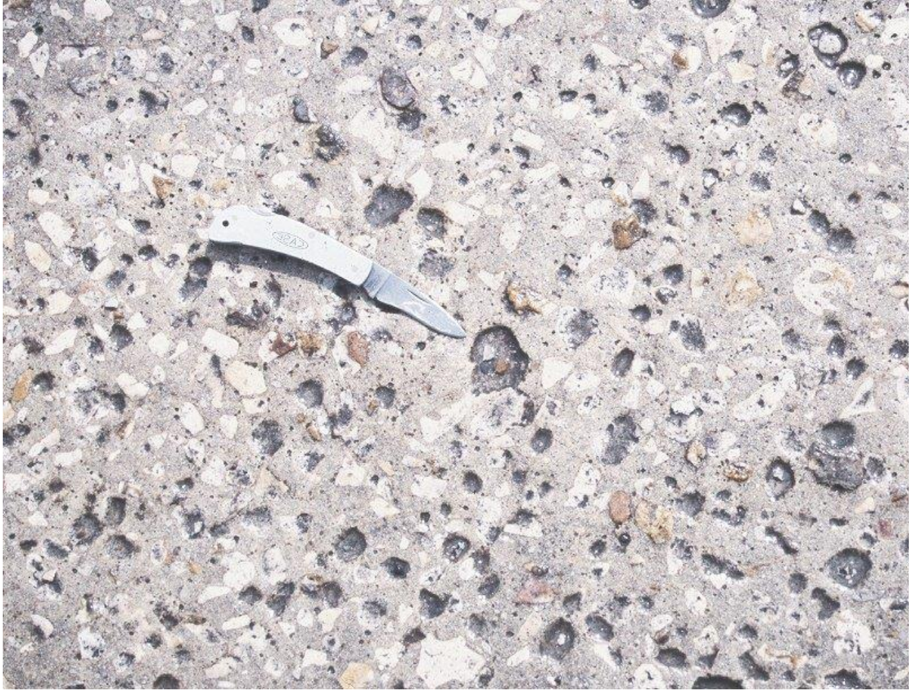
FIGURE 2. SURFACE DETERIORATION
