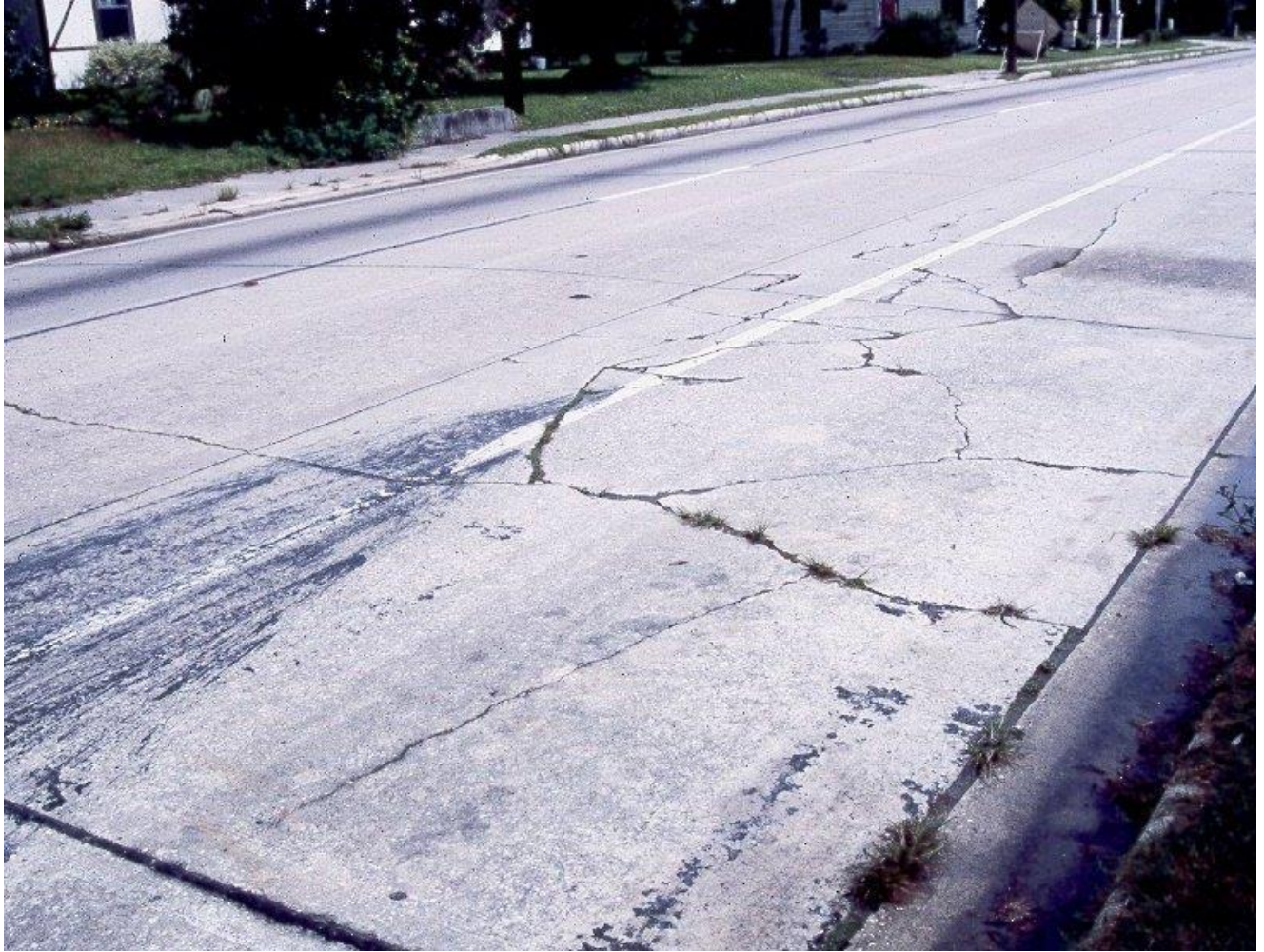
FIGURE 8. SHATTERED SLAB
