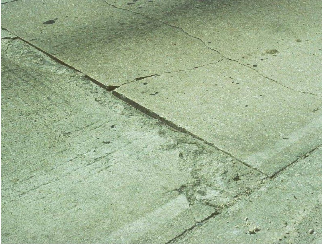
FIGURE 3. SPALLING
