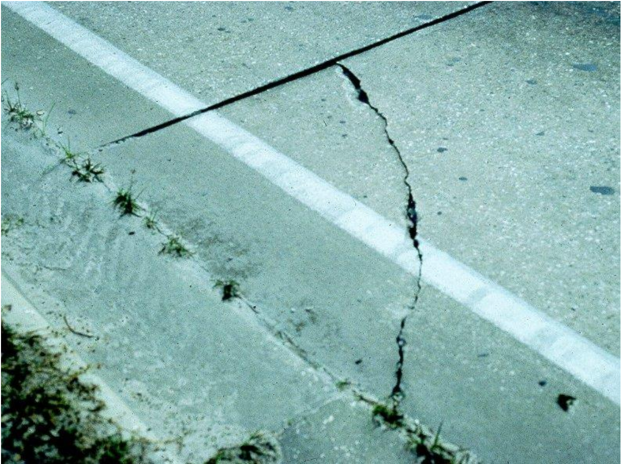
FIGURE 7. CORNER CRACKING
