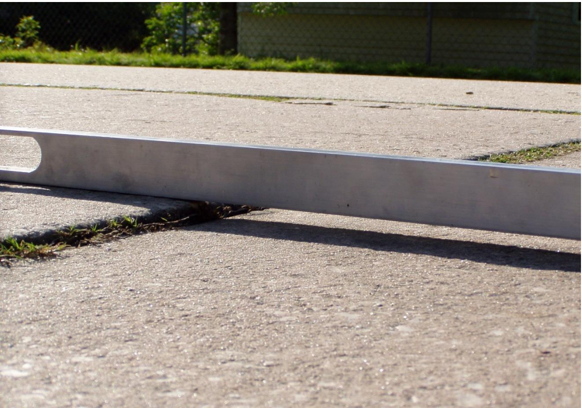
FIGURE 9. FAULTING
