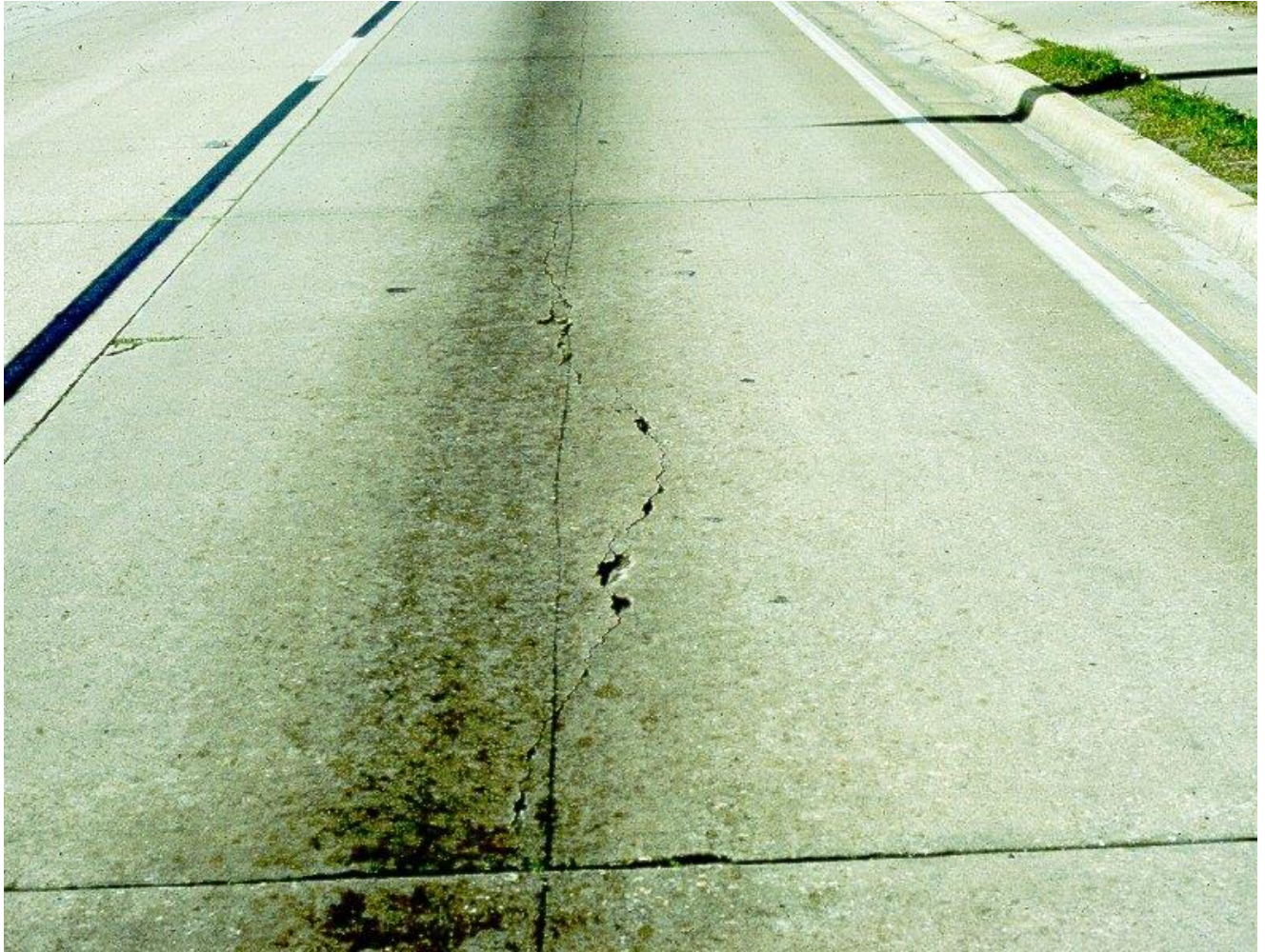
FIGURE 6. LONGITUDINAL CRACKING
