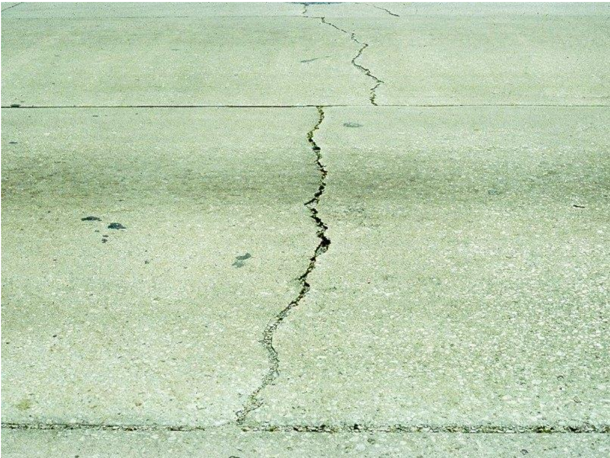
FIGURE 5. TRANSVERSE CRACKING
