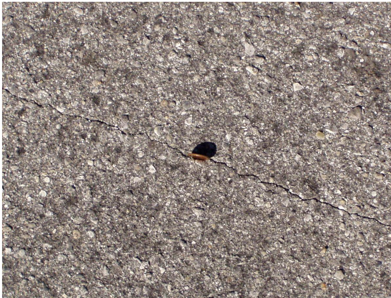
FIGURE 8. CLASS I CRACKING
