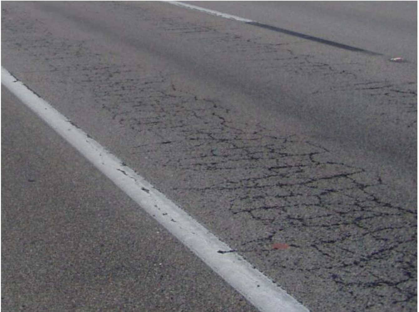
FIGURE 10. CLASS III CRACKING
