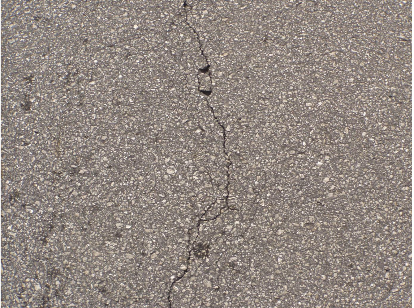
FIGURE 9. CLASS II CRACKING
