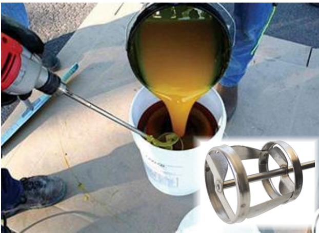
FIGURE 11 – Electric mixer with “Jiffy Mixer” attachment.
