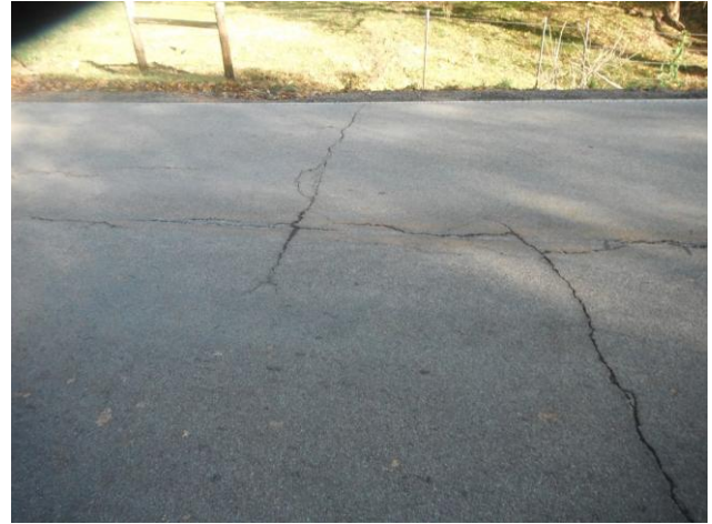
FIGURE 23 – Reflective cracking.
