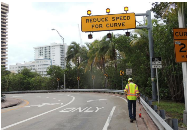
FIGURE 4 – HFST on Tight Curve before a Signalized Intersection.
