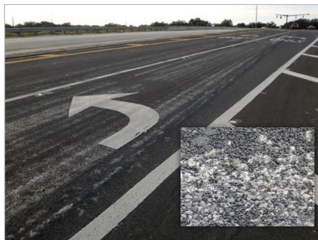
FIGURE 14 – Aggregate loss over uneven texture.
