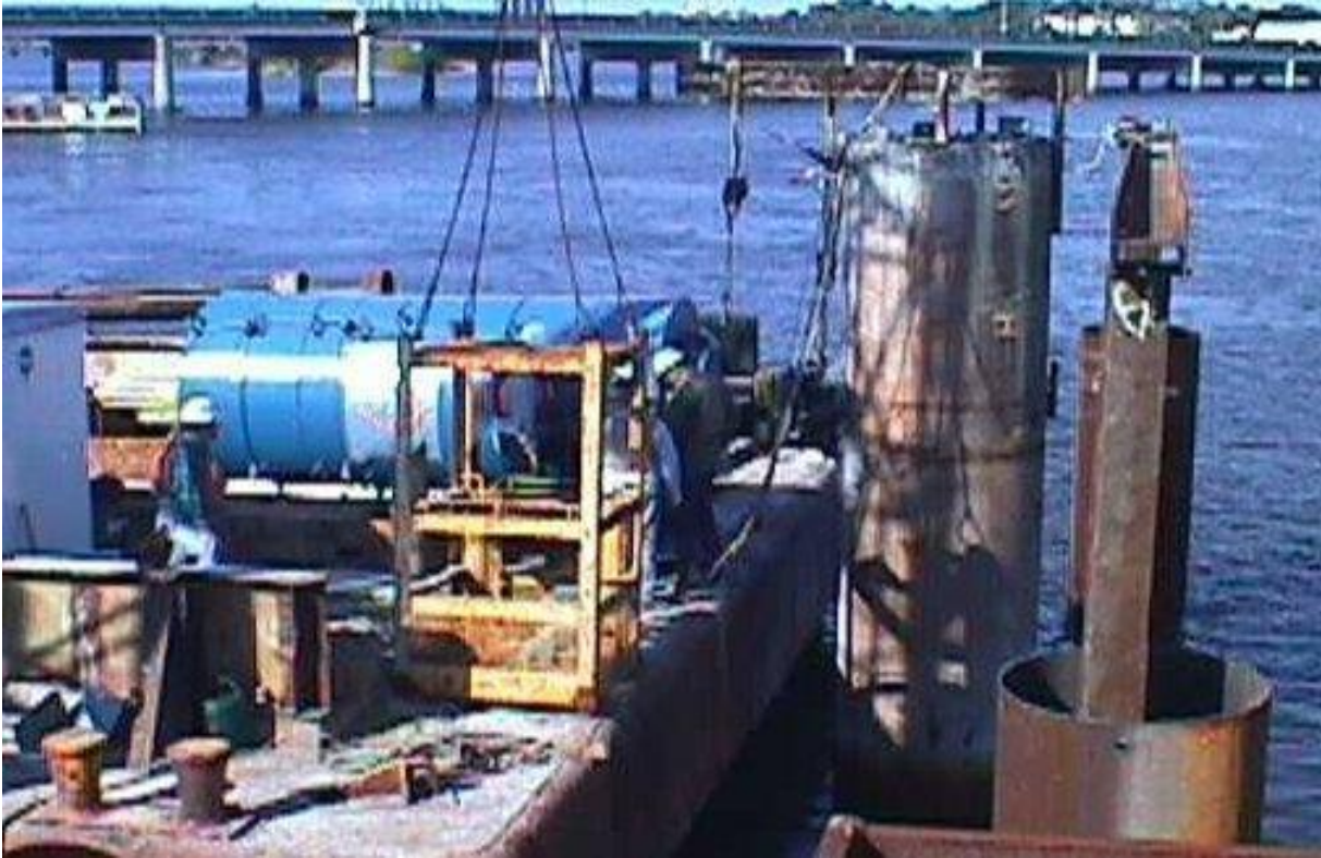
Figure 10-3: Lateral Statnamic Load Test
