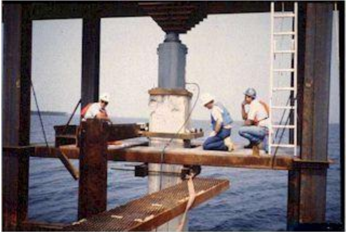
Figure 10-1: Static Load Test
