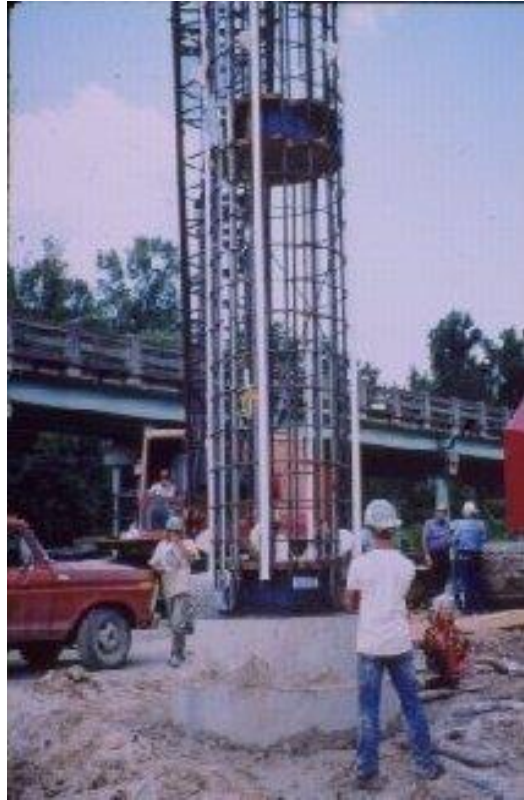
Figure 10-4: Osterberg Load Cells
