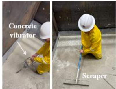
Leveling and vibrating to remove air bubbles
