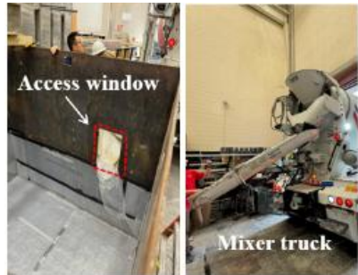
SL placement through access window
