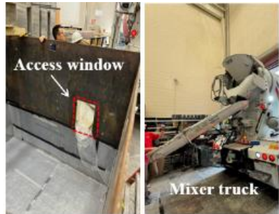
SL placement through access window
