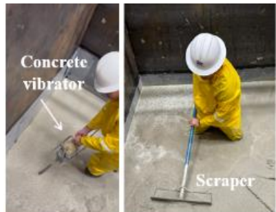
Leveling and vibrating to remove air bubbles
