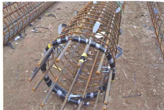
Protecting DFOS cables
