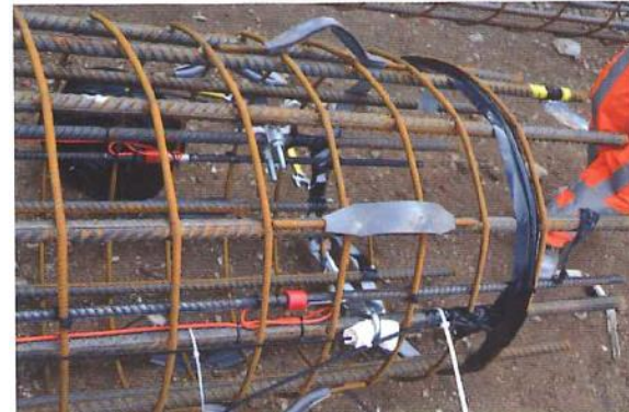
Pretensioning DFOS cables with cable clamps
