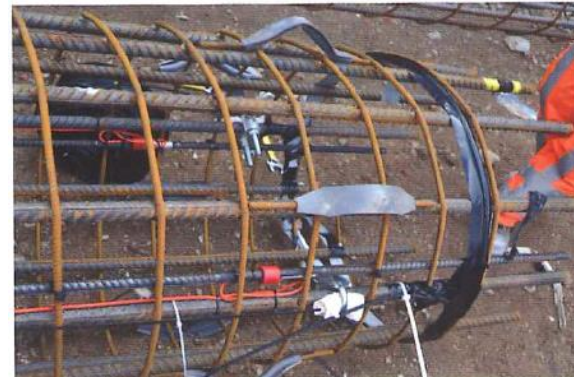
Pretensioning DFOS cables with cable clamps
