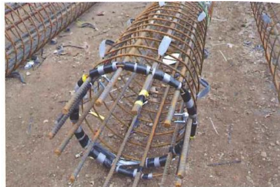
Protecting DFOS cables
