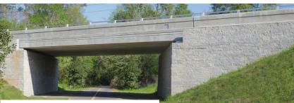
Single span <140 ft Abutment height<30 ft Service limit pressure 4 ksf
