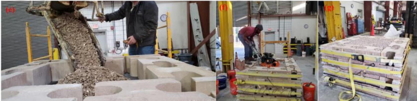
(a) Laying the face blocks, (b and c) Placing and compacting backfill, (d) Laying down geosynthetics, (e, f, and g) Repeat A-C to achieve final height
