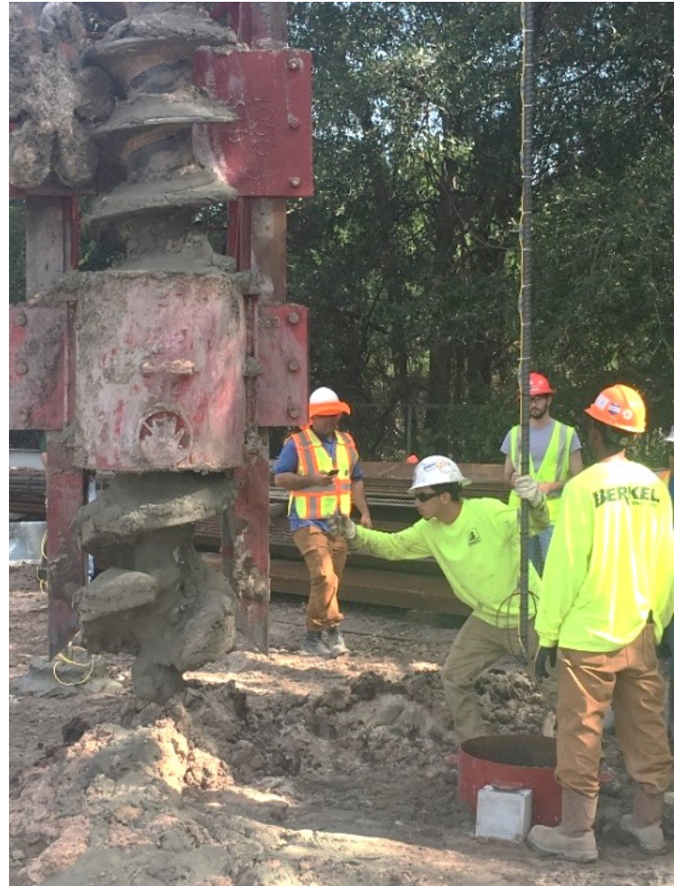
(left) soil clings to center stem (right) soil sits on auger flights
