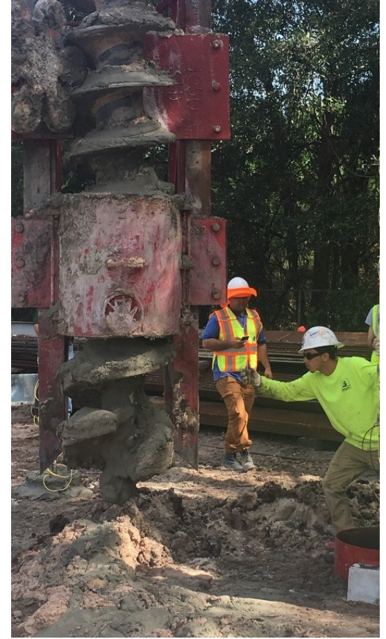
Soil cuttings sit on auger flights
