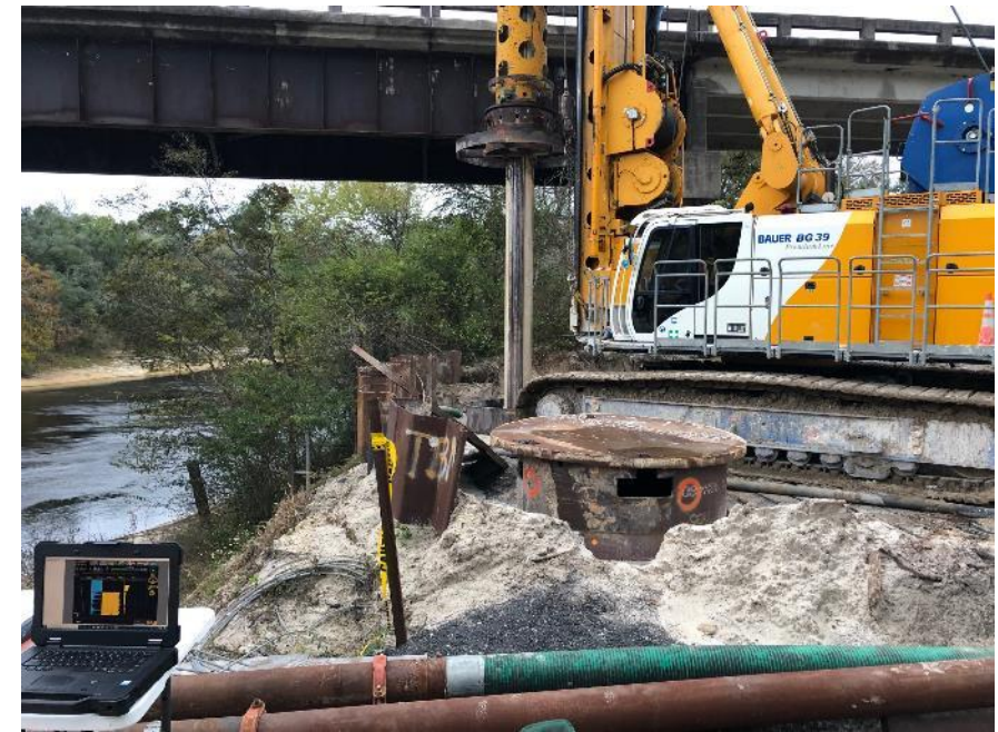
Bored Pile MWD – Construction QA/QC
