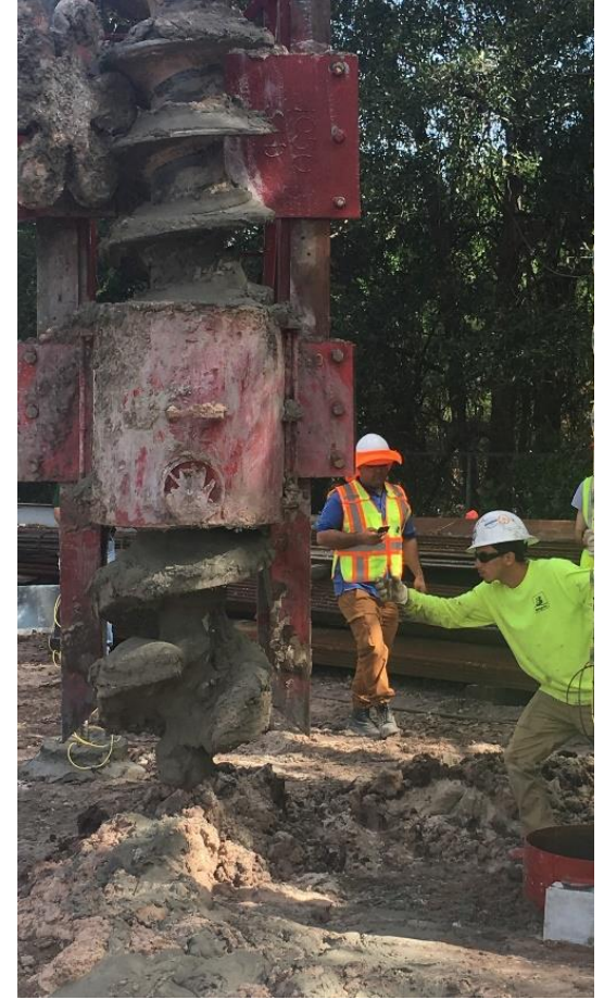
Soil cuttings sit on auger flights
