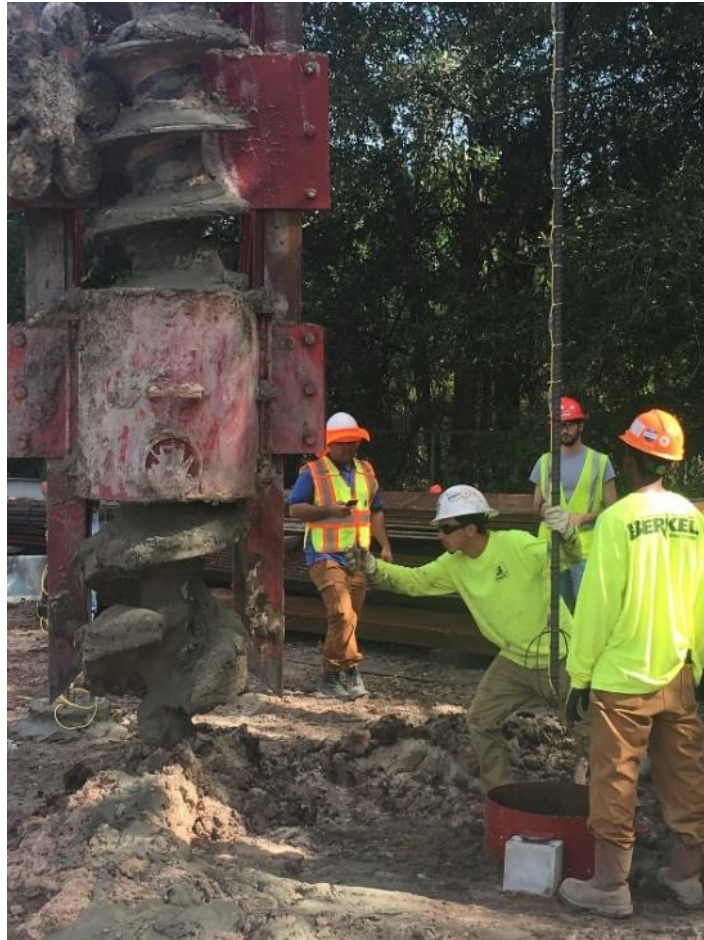
(left) soil clings to center stem (right) soil sits on auger flights
