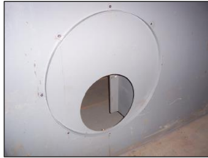
Entry port for “void” installation and sediment transport (BELOW)
