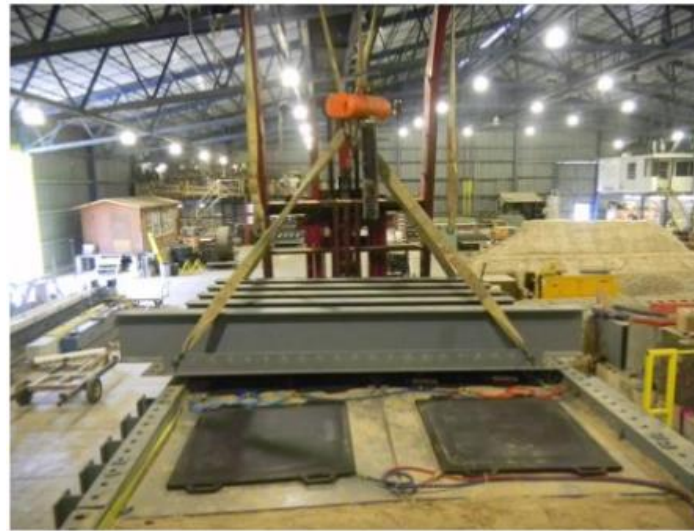
(LEFT) Installation of I-Beam roof for reaction force of airbags and overburden simulation
