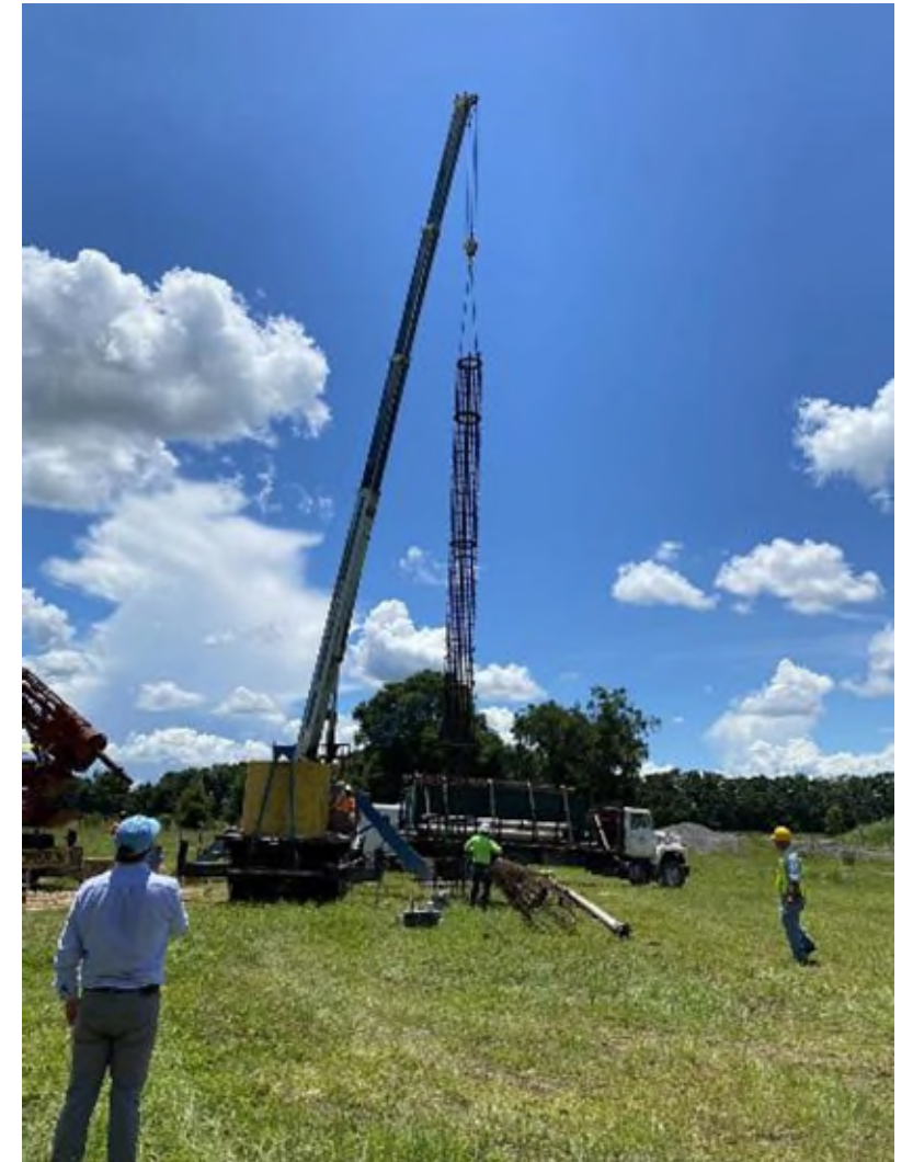
Rebar Cage Installation
