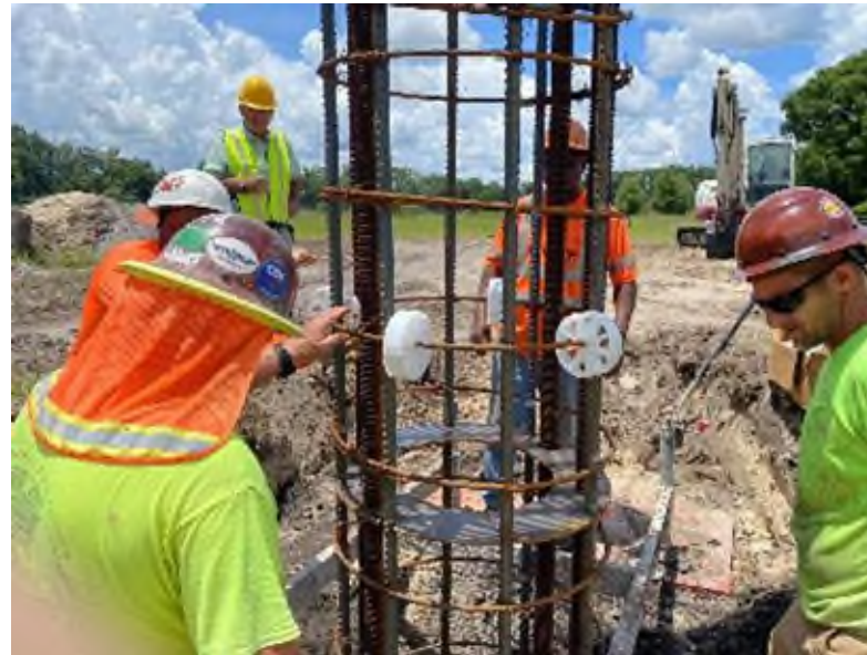
Rebar Cage Placement
