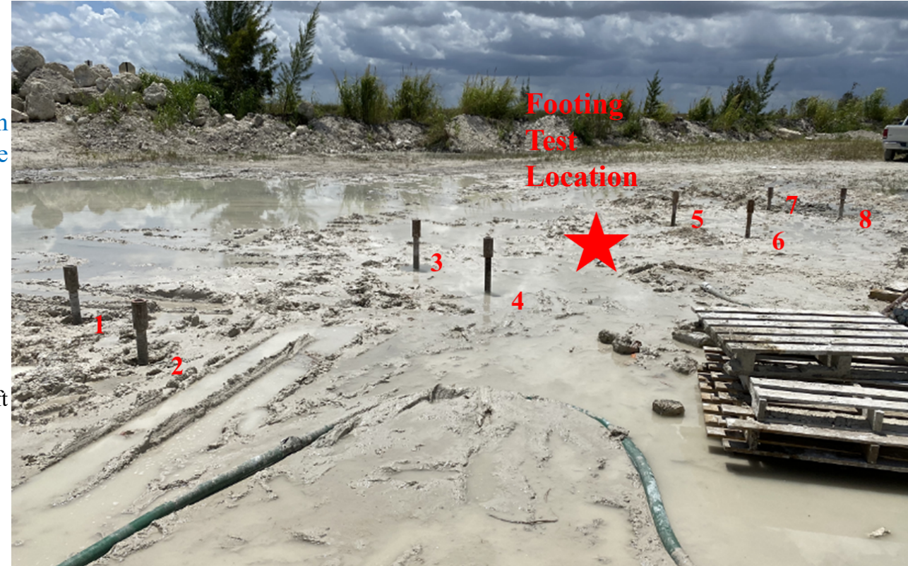
Drilling and Micro-piles Installation (H2R)
