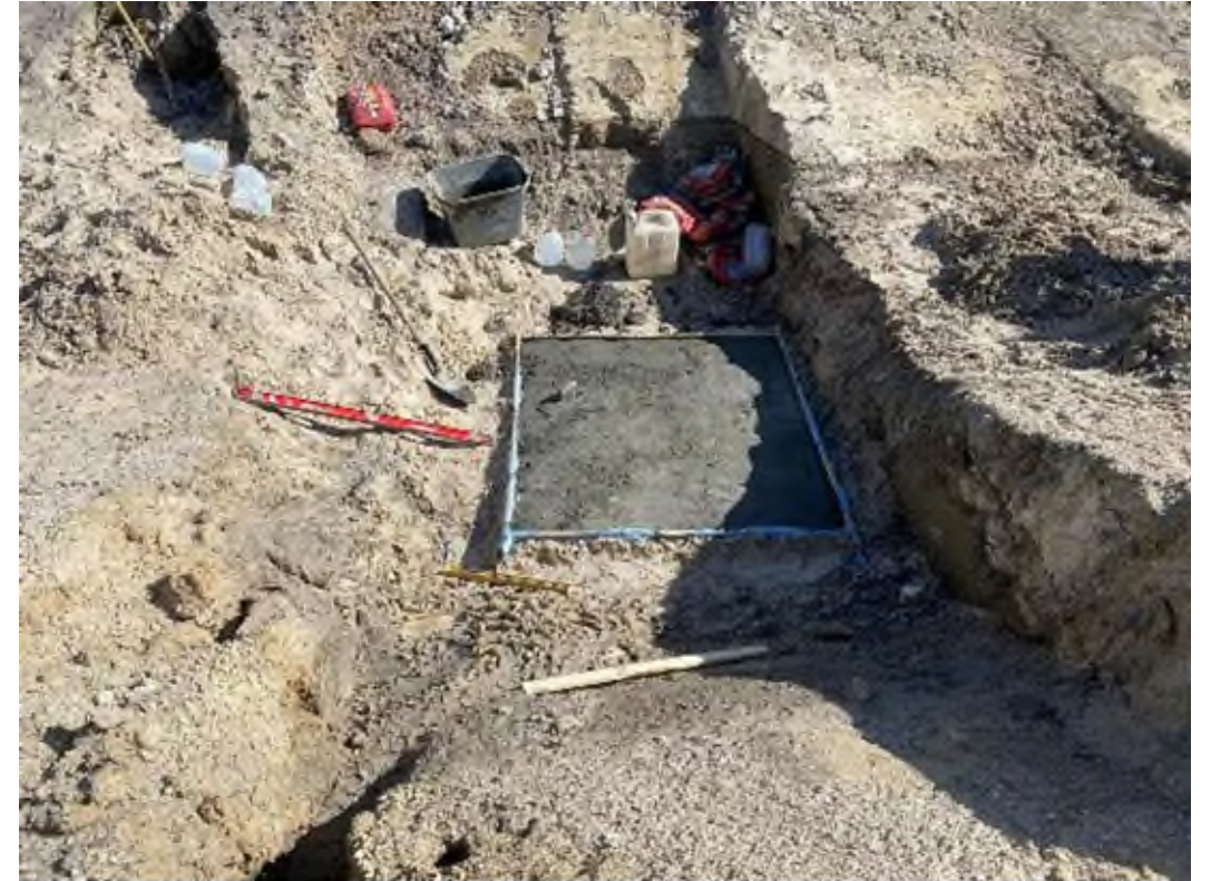
Leveled Concrete at Footing Location
