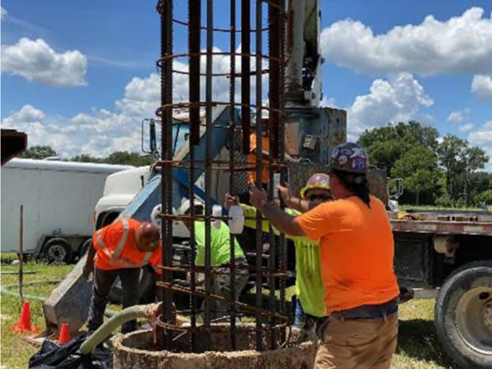
Rebar Cage Installation
