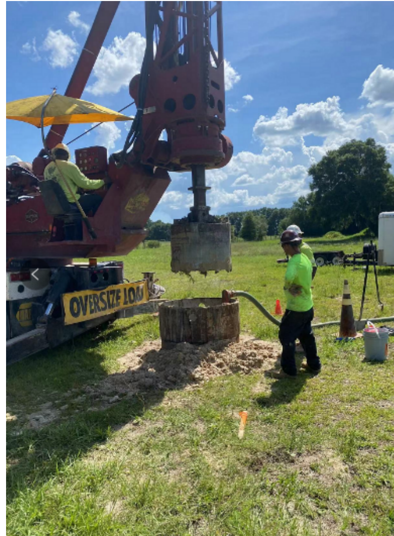
Bailing Bucket to clean the hole
