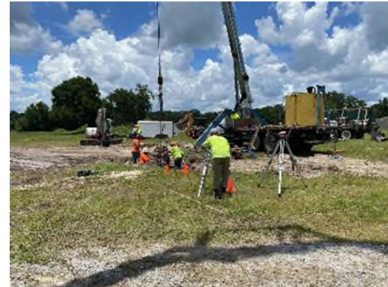
Leveling Shafts
