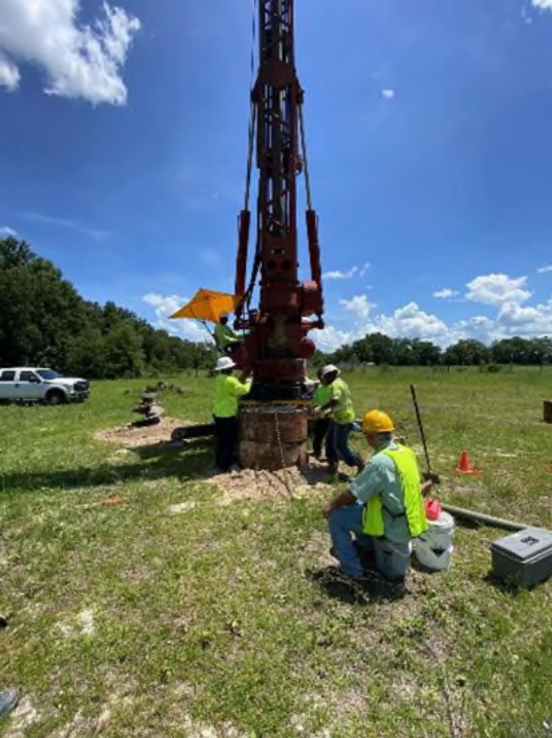
Casing Placement
