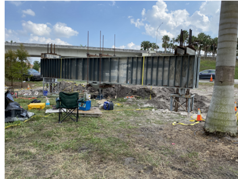
Hydraulic Jack and Load Cell Setup
