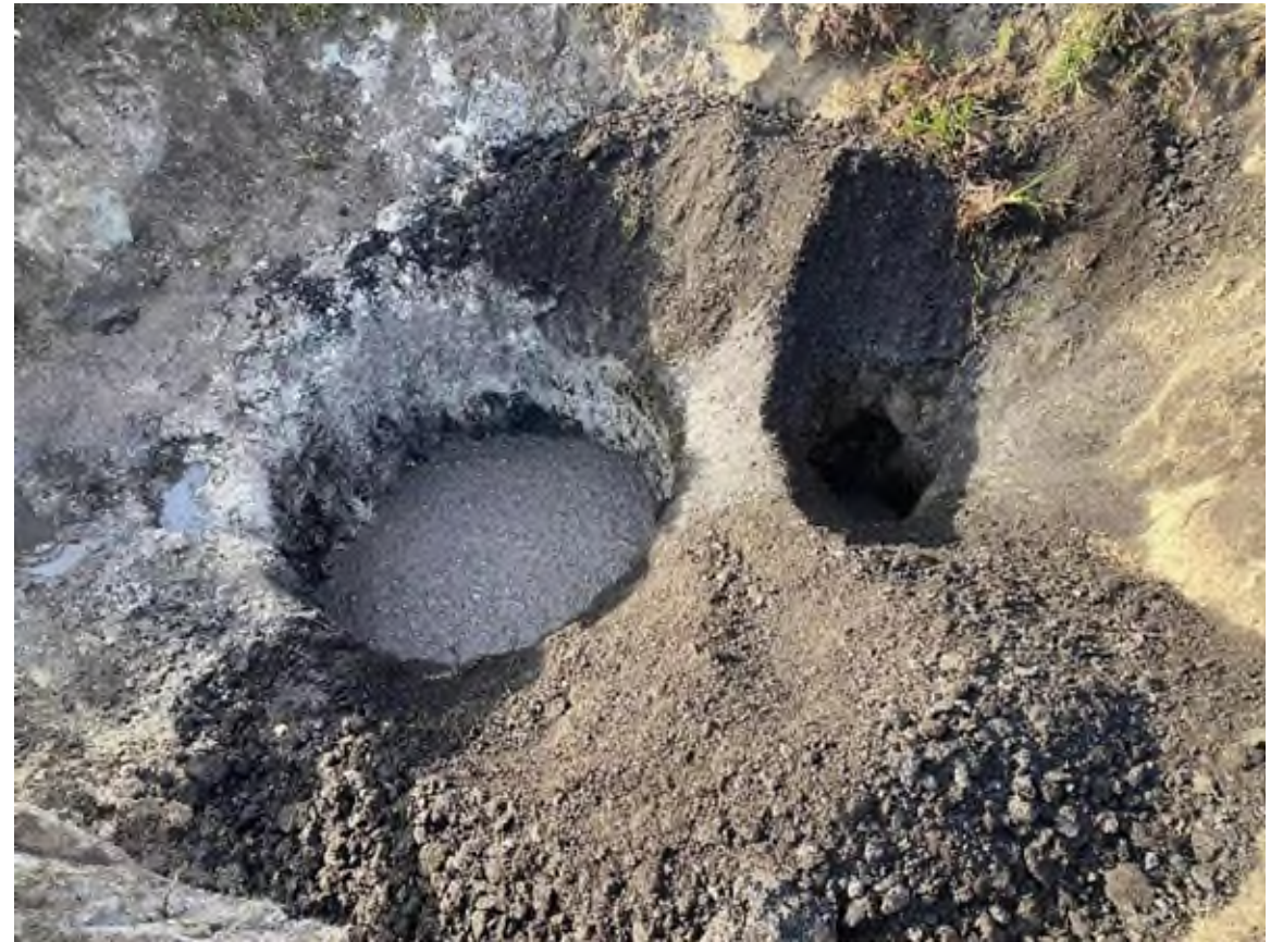
Fill the drilling hole and sinkhole with asphalt
