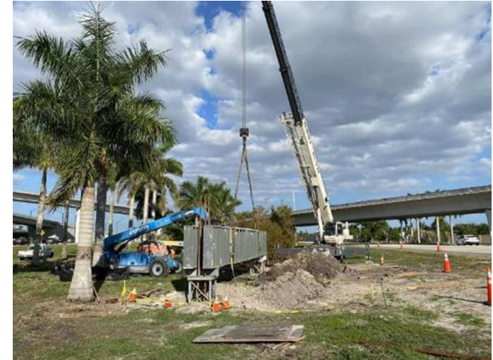
Installation of Girders
