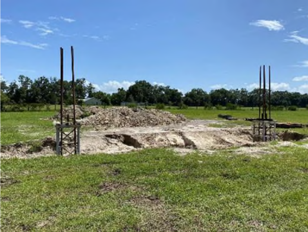
Threaded Rods and Stands Placement
