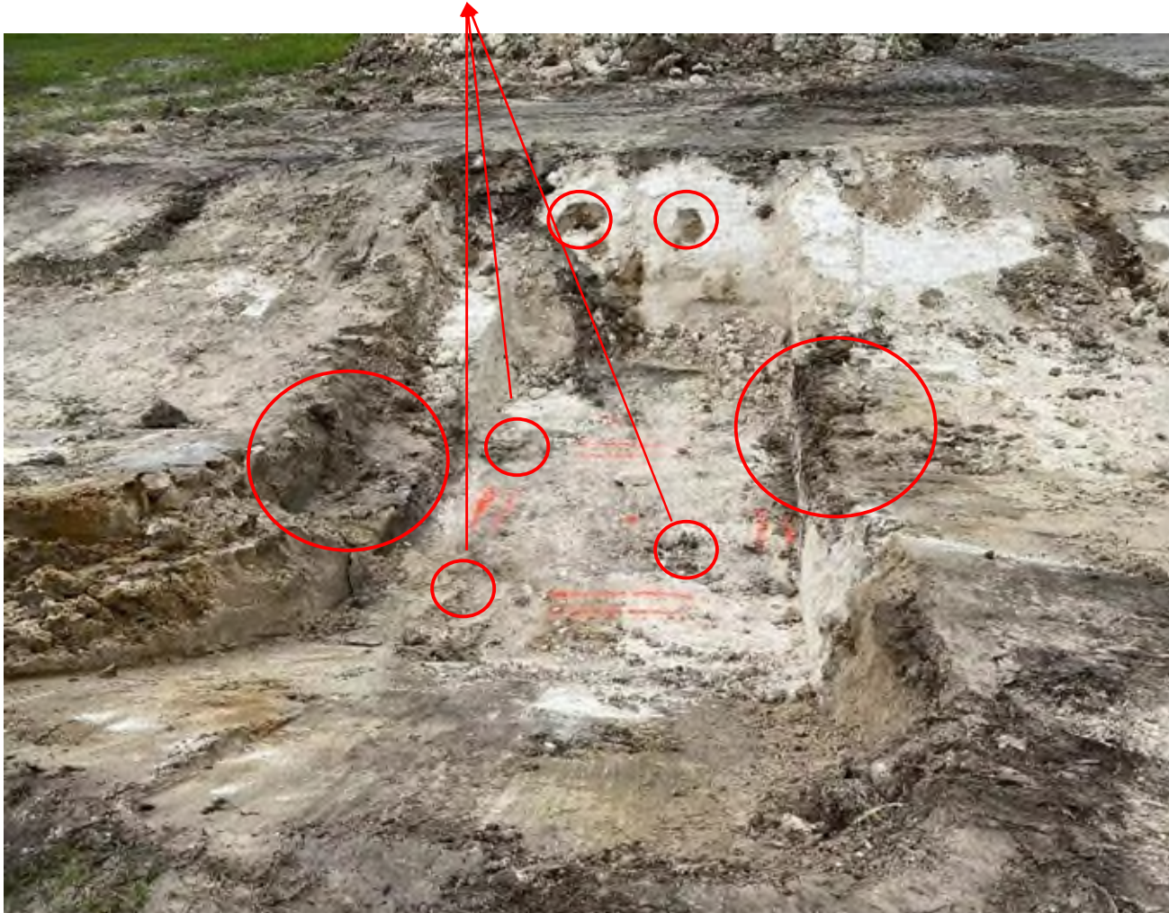
Top of Rock Surface at 5 ft depth
