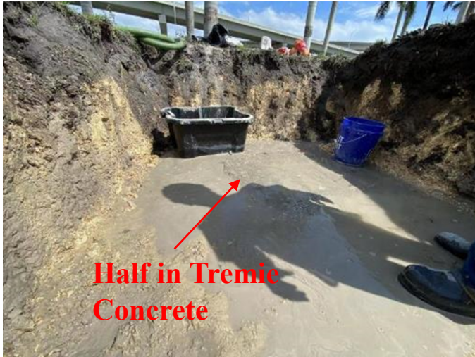
Fasting Setting Concrete for footing placement
