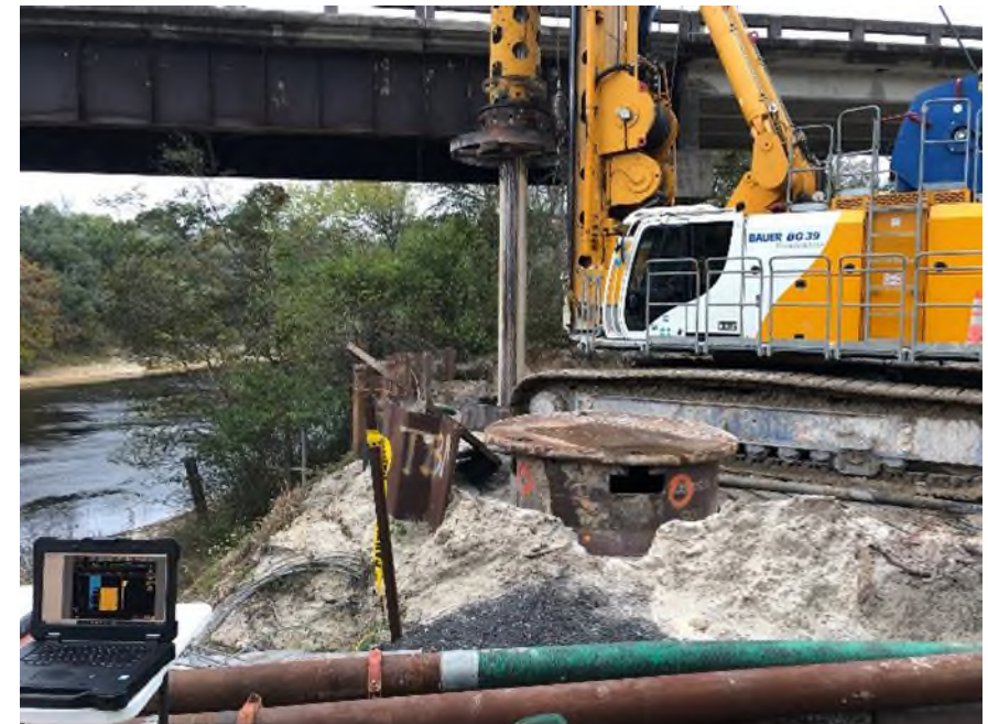
Bored Pile MWD – Construction QA/QC
