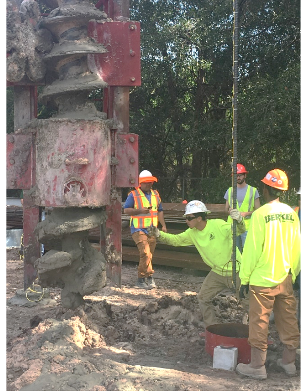
Soil cuttings sit on auger flights
