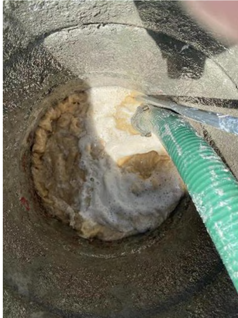
Mix with ASTM C494 Type D Retarder admixture and ASTM C494 Type F Superplasticizer admixture
