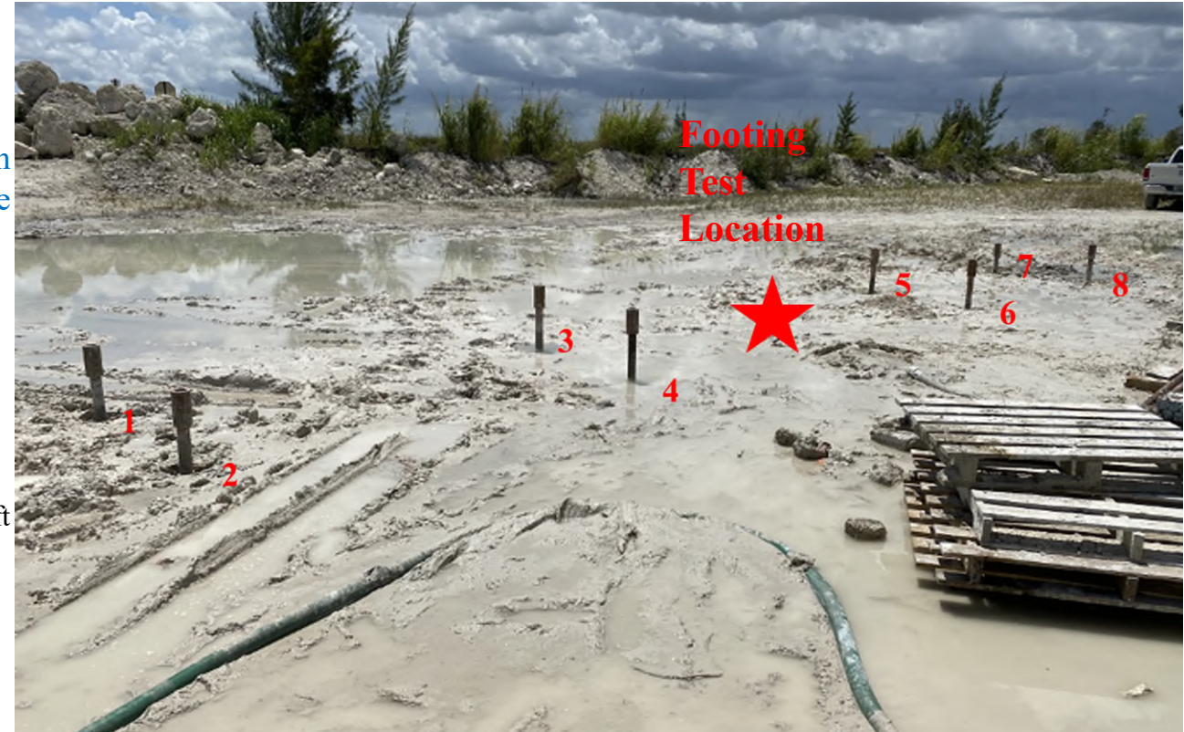
Drilling and Micro-piles Installation (H2R)
