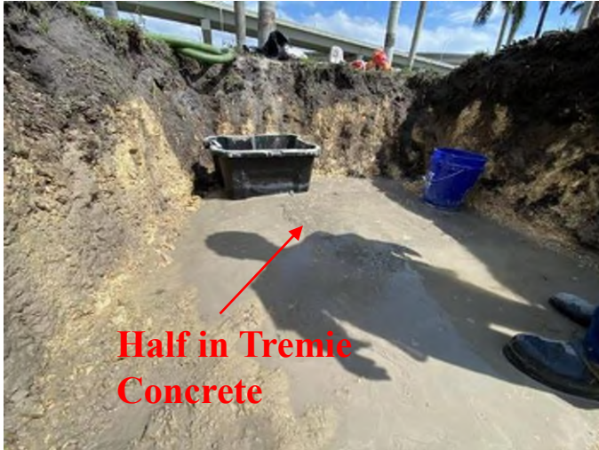
Fasting Setting Concrete for footing placement
