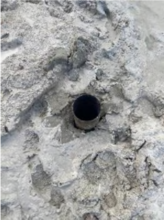
Drill with Polymer Mud System – Tight Holes
