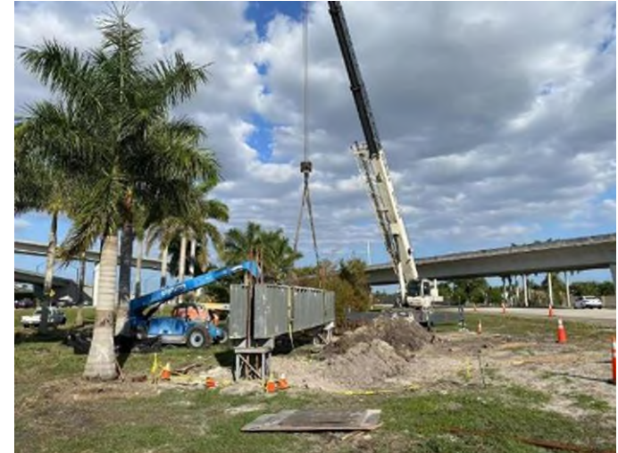
Installation of Girders
