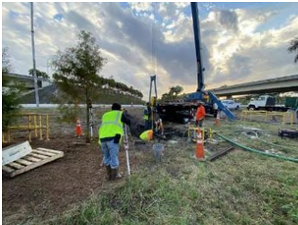
Alignment with West Shaft
