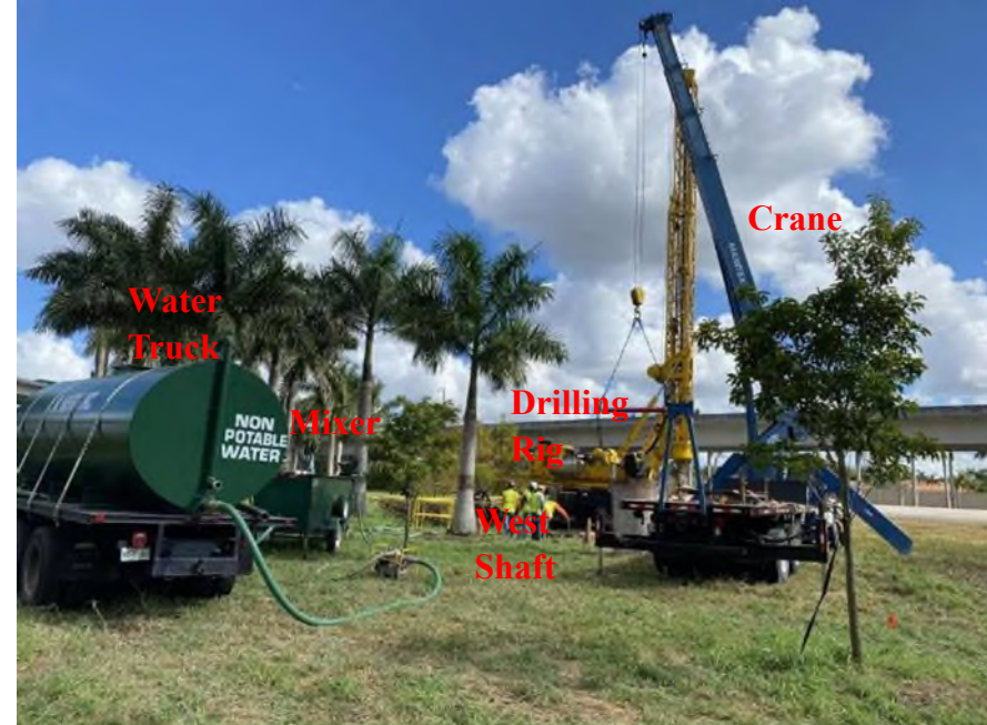
Drilling Setup
