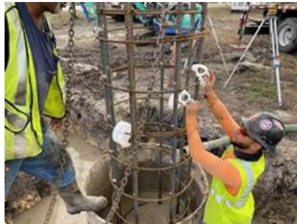
Placement for Rebar Cage
