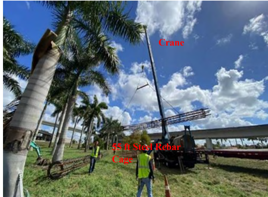
Steel Rebar Cage
