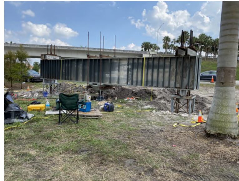
Hydraulic Jack and Load Cell Setup
