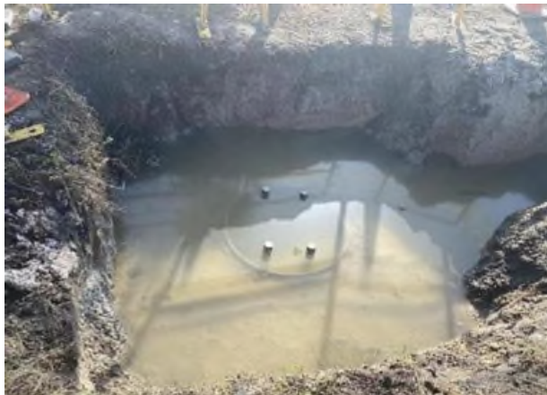
Picture of East Shaft after two days
