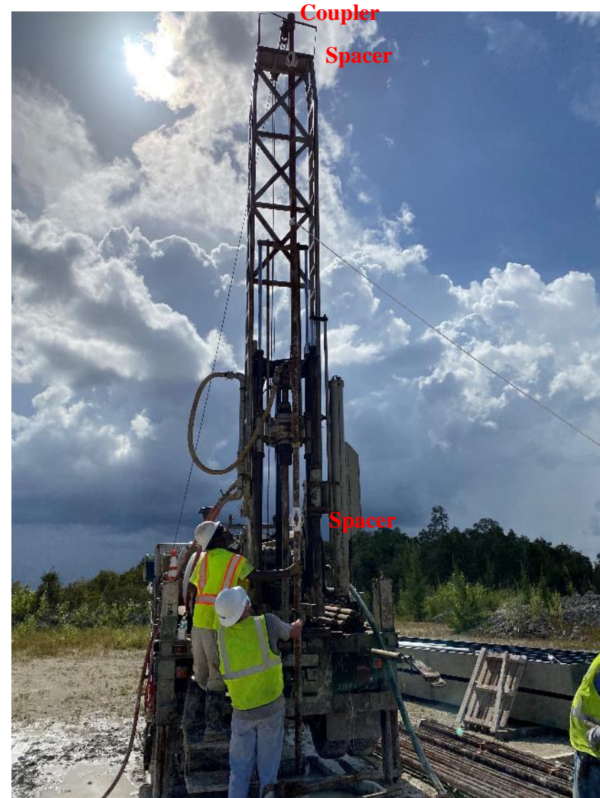
Placement of 36 ft long #18 Grade 80 Threaded Rebars
