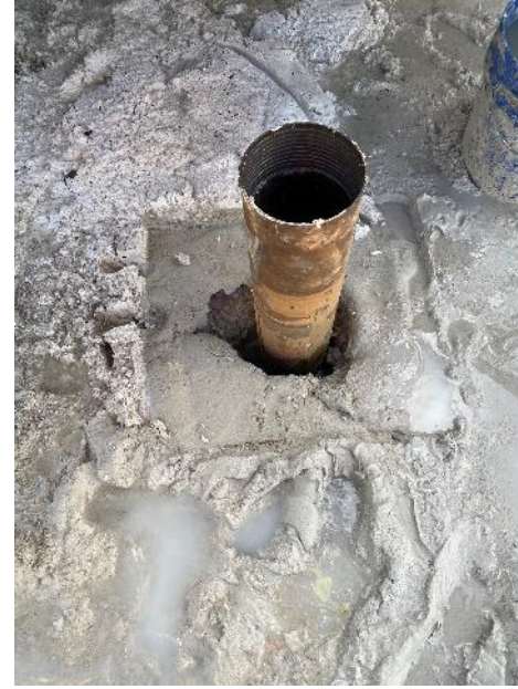
Drill with Clear Water – Loose Holes
