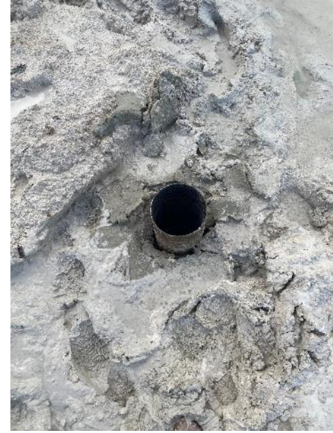
Drill with Polymer Mud System – Tight Holes
