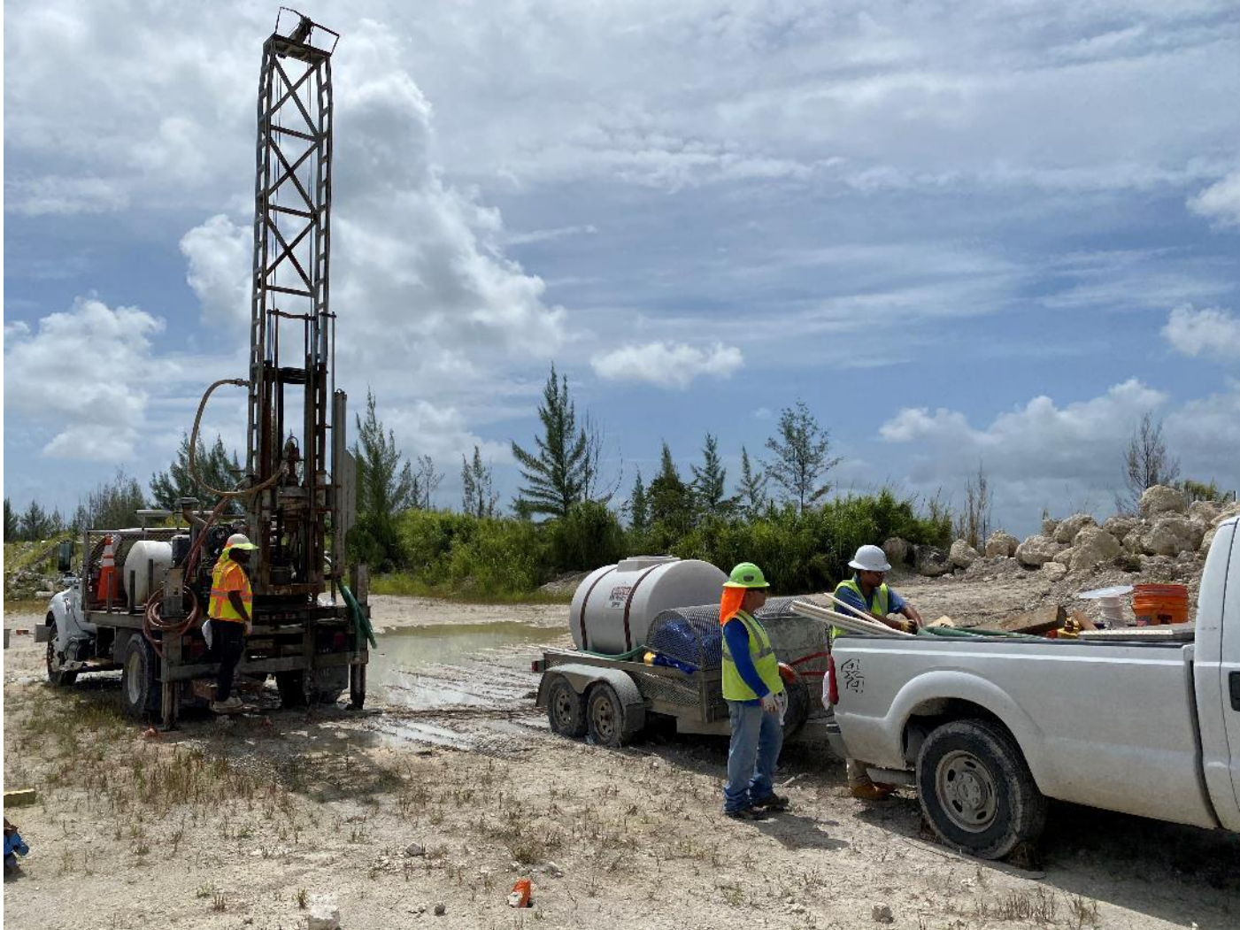
Drill Rigs and Water Tank
