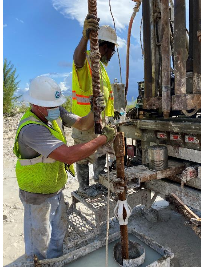
Placement of 20 ft long #18 Grade 80 Threaded Rebars
