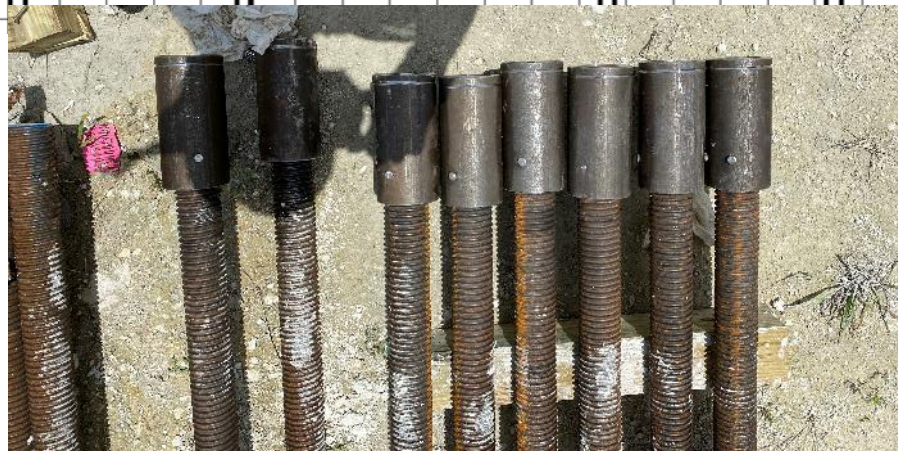
Bolts on Couplers to prevent rotation of bottom threaded rebar when unscrewing
