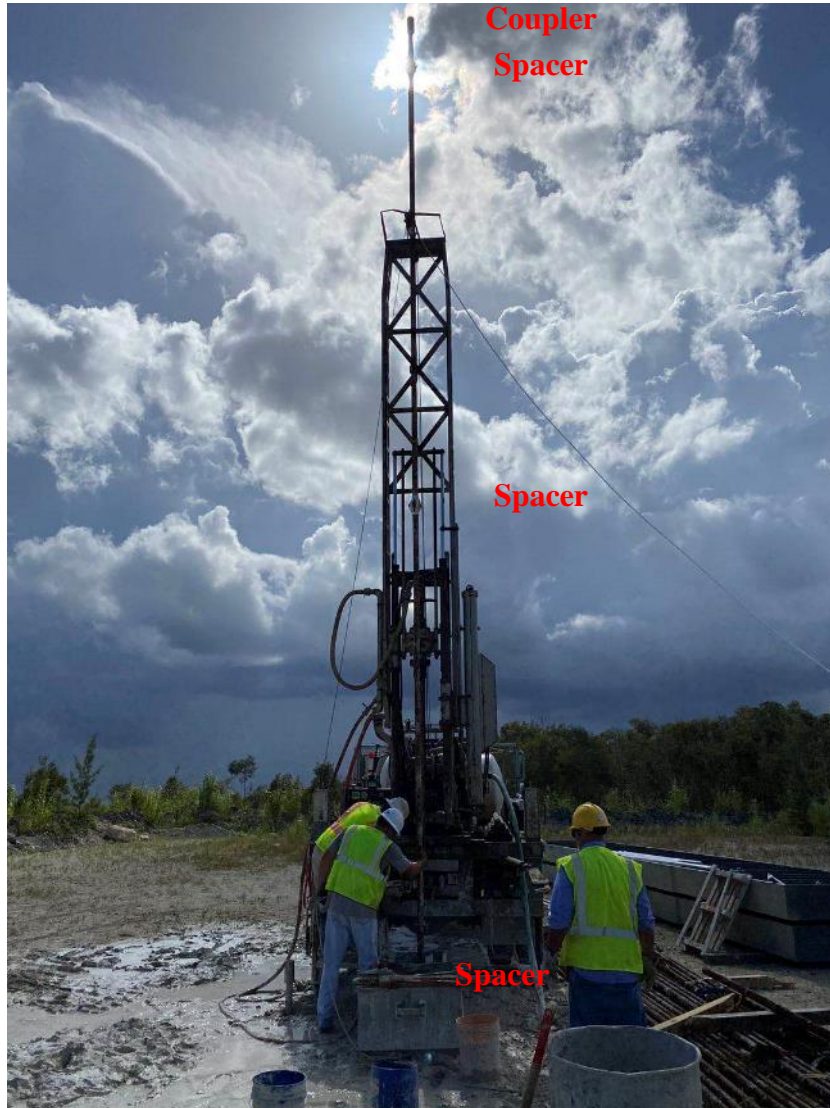
Placement of 36 ft long #18 Grade 80 Threaded Rebars
