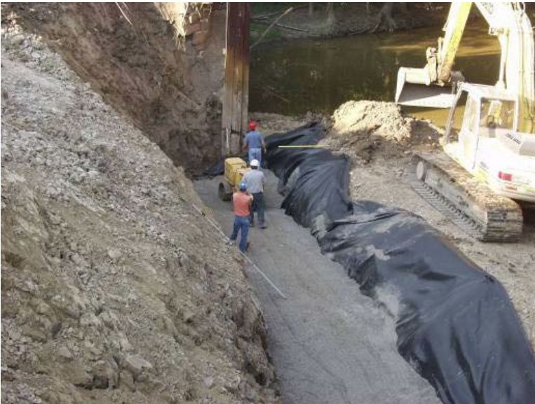
Encapsulation of fill in RSF (Adams and Nicks, 2018)
