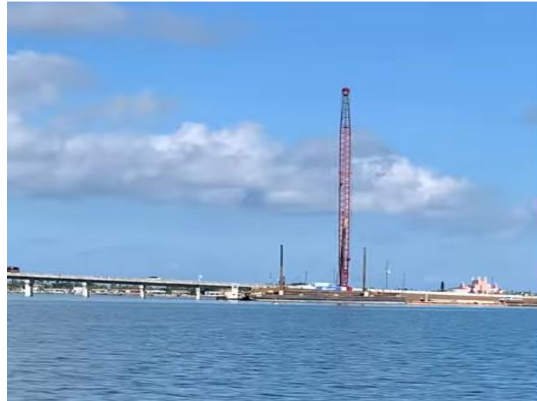
Bayway E Pile Rig
