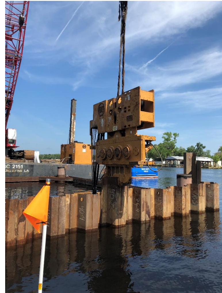
Dunn's Creek Sheet Piles
