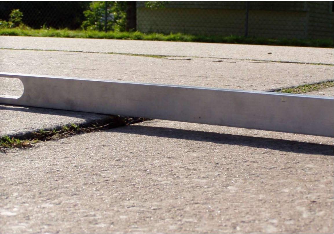
FIGURE 9. FAULTING
