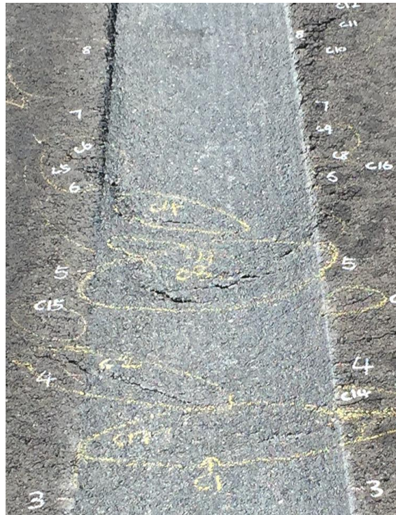
Figure 7. The unbonded section after the application of 0.6 million ESALs
