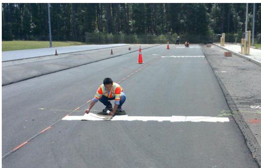
Figure 2. Preparation for measuring tack coat residual rate
