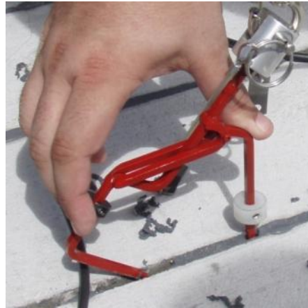
FIGURE 6 Inserting the hook through the sealant
