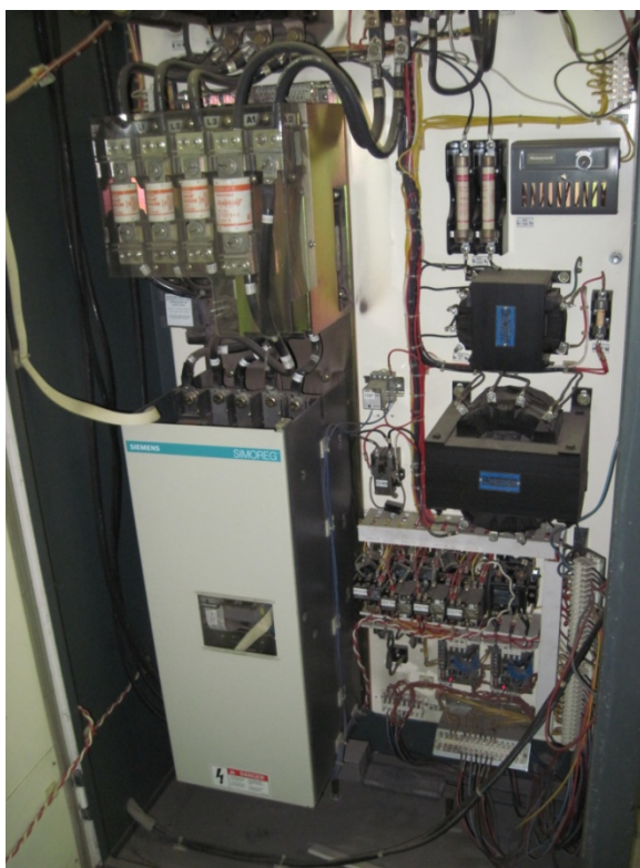
Figure 2.8.3.13.7.6-1 – DC drive controller
