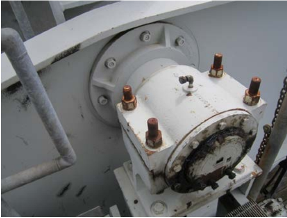
Figure 2.8.2.3.3-1 – A bascule bridge split sleeve type trunnion bearing
