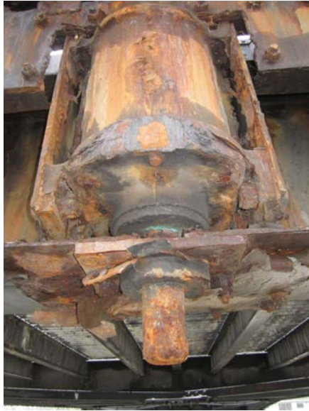
Figure 2.8.2.5.1-1 – Buffer cylinder and piston rod; note that the buffer is heavily corroded and not functional
