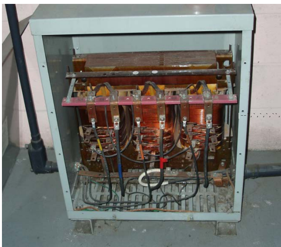
Figure 2.8.3.7.3.1-1 – Air-cooled transformer
