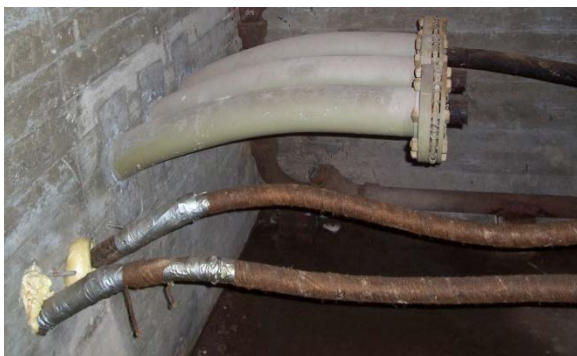
Figure 2.8.3.6.1-1 – Deterioration of electrical cables
