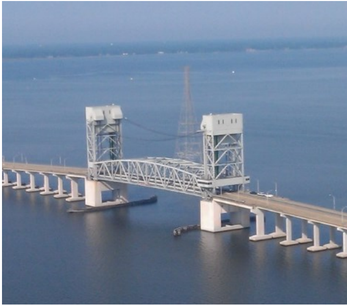
Figure 1.3.3.1-1 – Tower-drive vertical-lift bridge
