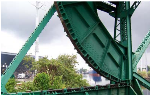
Figure 2.8.2.11.1.2-1 – Segmental girder and tread plate of track girder (the girder is embedded in the pier concrete)
