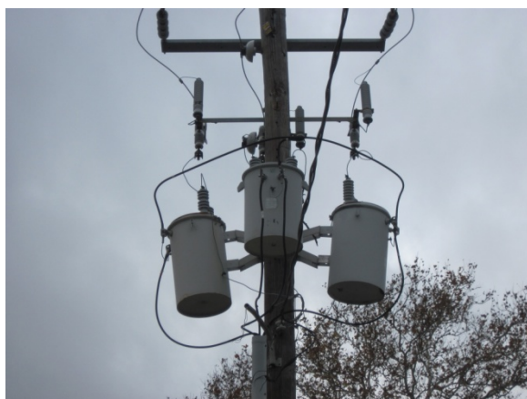
Figure 2.8.3.7-1 – Pole mounted transformers
