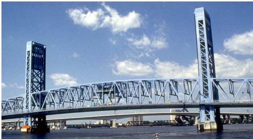
Figure 1.3.3.1-3 – Span-drive vertical-lift bridge
