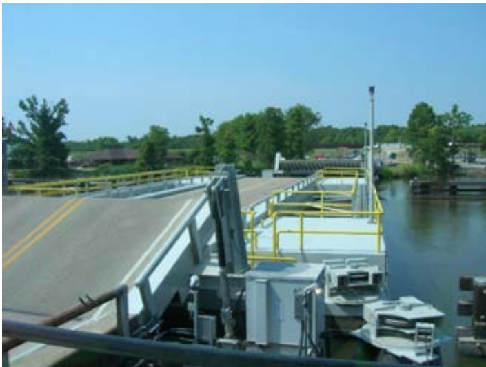
Figure 1.3.4-1 – Pontoon swing-span bridge with wire rope operation, Louisiana
