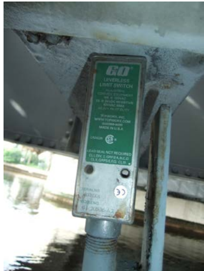
Figure 2.8.3.13.3.1-5 – A proximity limit switch
