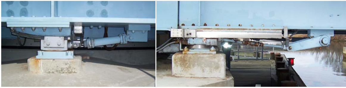
Figure 2.8.2.11.2.4-6 – Live load shoes on a swing-span bridge
