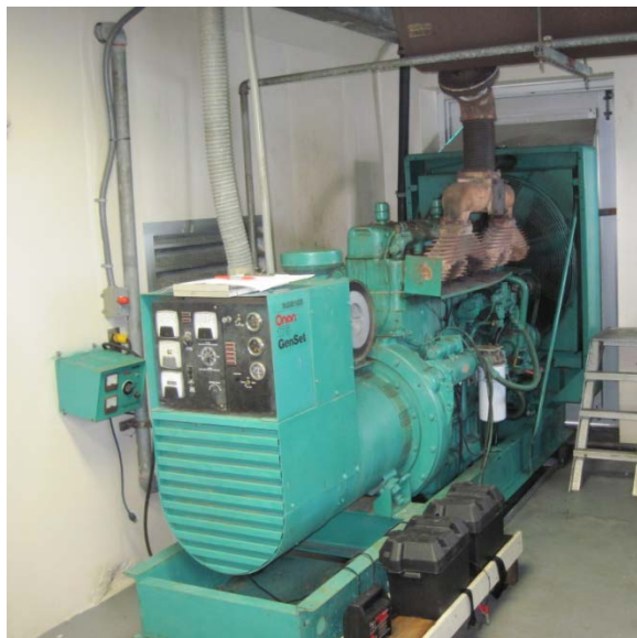
Figure 2.8.3.7.2-1 – An automated generator
