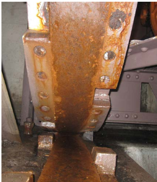
Figure 2.8.2.11.1.2-2 – Segmental girder and tread plate of track girder
