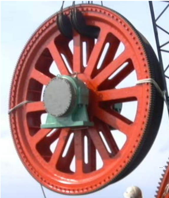
Figure 2.8.2.3.3-2 – A large diameter roller bearing pillow block on a vertical-lift bridge
