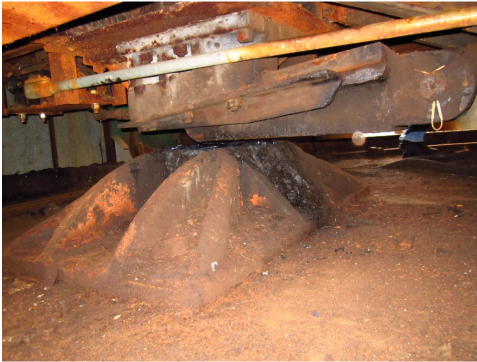
Figure 2.8.2.11.2.4.1-1 – Improper bearing of live load shoe
