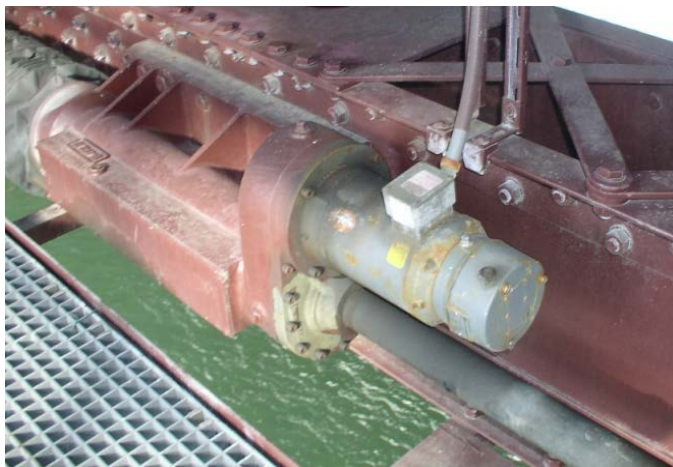
Figure 2.8.3.3-1 – A span lock motor
