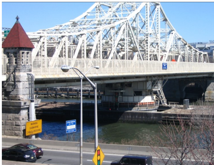
Figure 1.3.2.1-5 – Rim bearing swing-span
