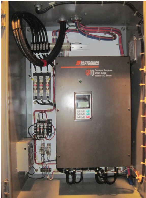
Figure 2.8.3.13.7.4-1 – A motor control center with integral VFD controller
