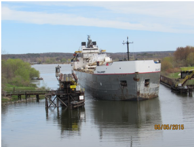
Figure 4.5.2-2 – Navigation problems created by movable span location
