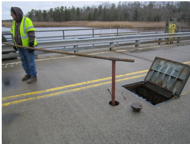
Figure 2.8.2.8.2-1 – Manual drive on a swing bridge
