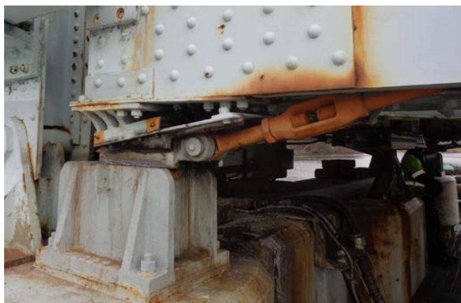
Figure 2.8.2.11.2.4-2 – End wedge, crank, and turnbuckle
