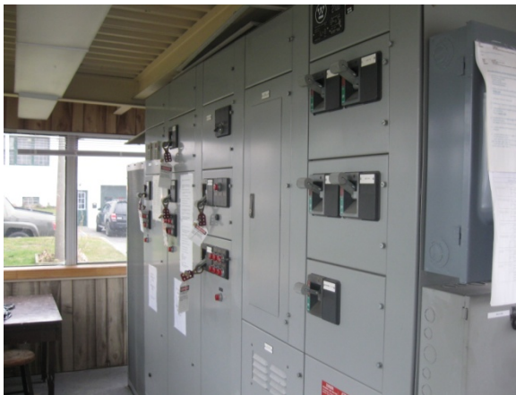
Figure 2.8.3.4-2 – Motor control center
