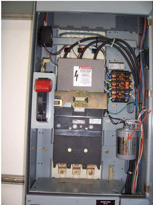
Figure 2.8.3.13.8.1-1 – Incoming power surge suppressor
