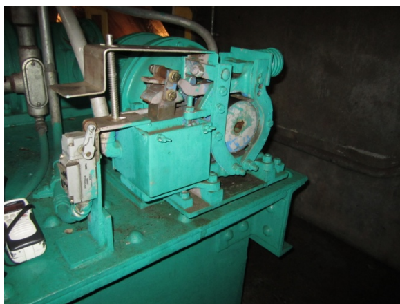
Figure 2.8.3.5.2-2 – Solenoid type brake
