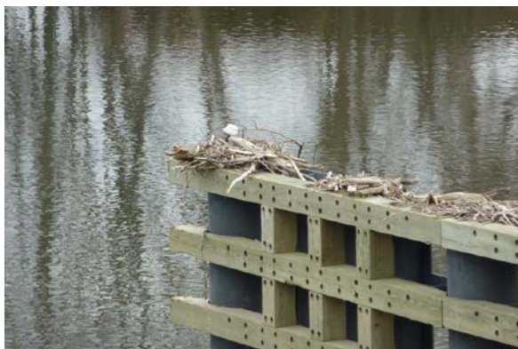
Figure 2.8.1.5.3-1 – Debris accumulation on fender system and damage to navigation lights
