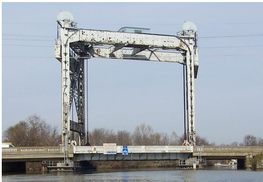
Figure 1.3.3.1-5 – Connected-tower vertical-lift bridge
