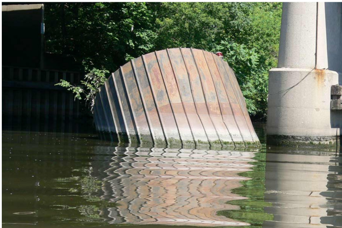
Figure 2.8.1.5.4-4 – Damaged pier protection cell
