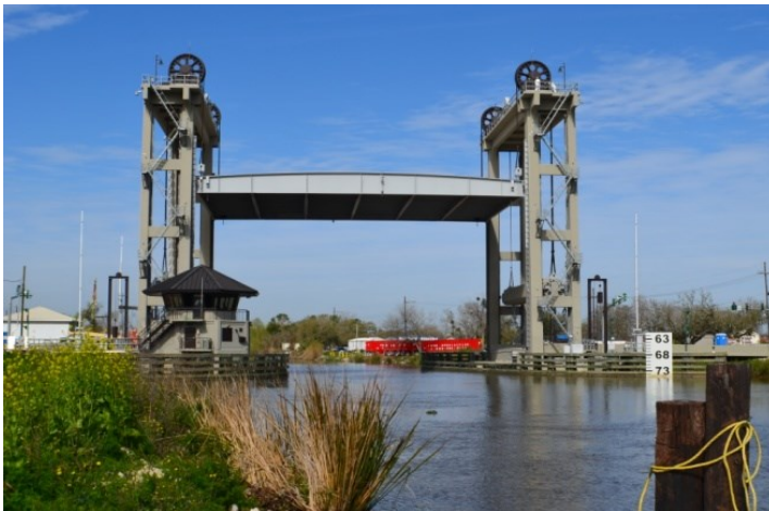
Figure 1.3.3-1 – Vertical-lift with concrete towers and plate girders
