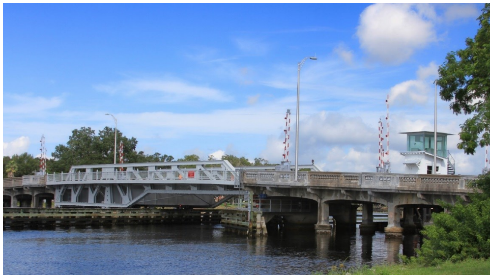
Figure 1.3.2-2 – Bob-tail swing-span bridge
