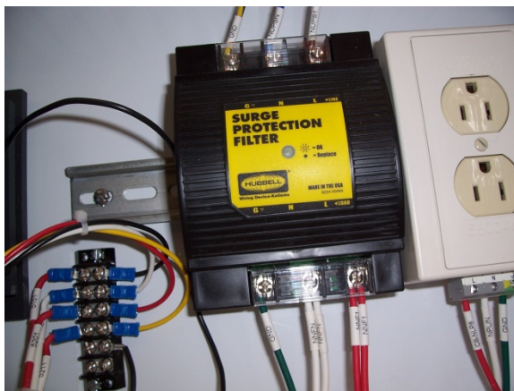
Figure 2.8.3.13.8.1-2 – PLC power surge suppressor
