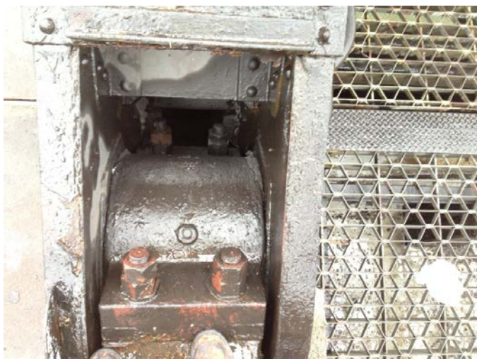
Figure 2.8.2.3.3-3 – Trunnion bearing on a Strauss heel trunnion bascule bridge
