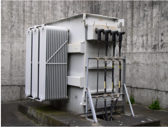
Figure 2.8.3.7.3.2-1 – A liquid-filled transformer
