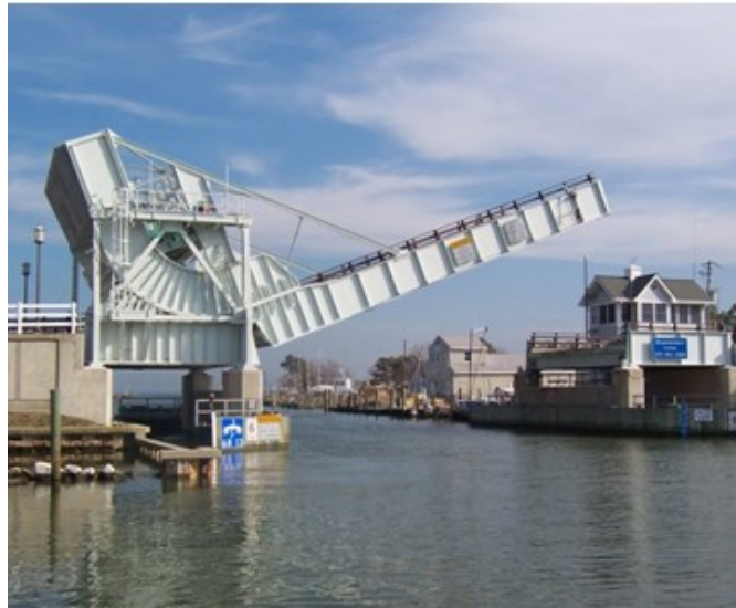
Figure 1.3.1.1-3 – Rolling-lift single-leaf bascule
