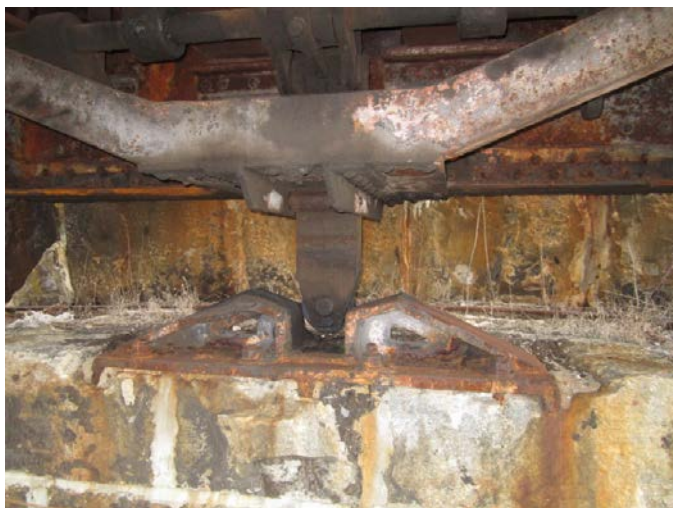
Figure 2.8.2.11.2.5.1-1 – Latch bar engaged in pocket
