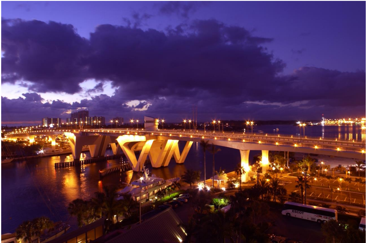
17 th Street Bridge over Intracoastal Waterway, Fort Lauderdale
