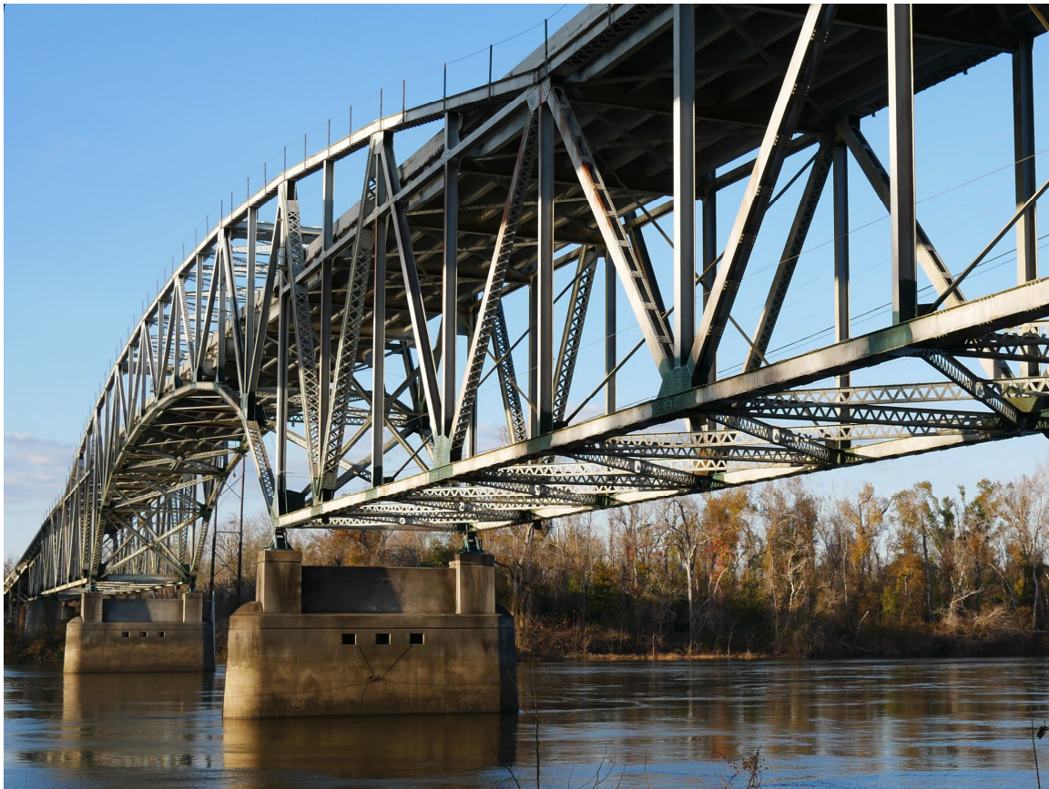
Trammel Bridge, SR20 westbound over Apalachicola River
