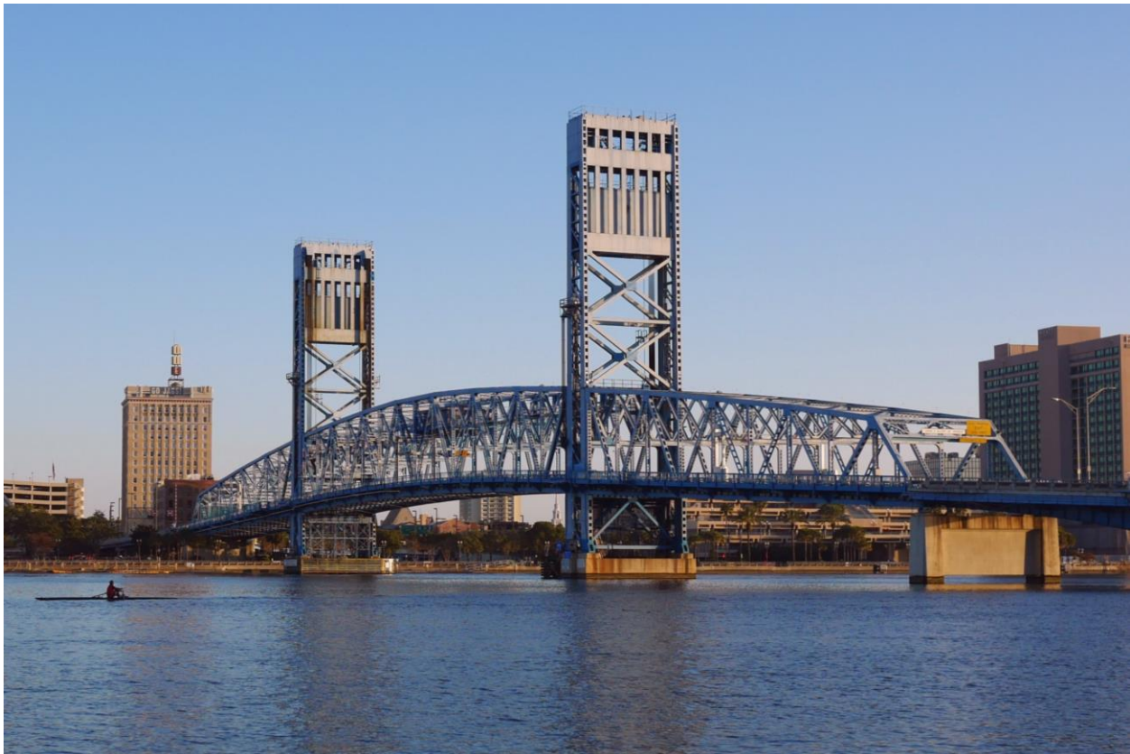
John T. Alsop Bridge, Main Street over St. Johns River in Jacksonville
