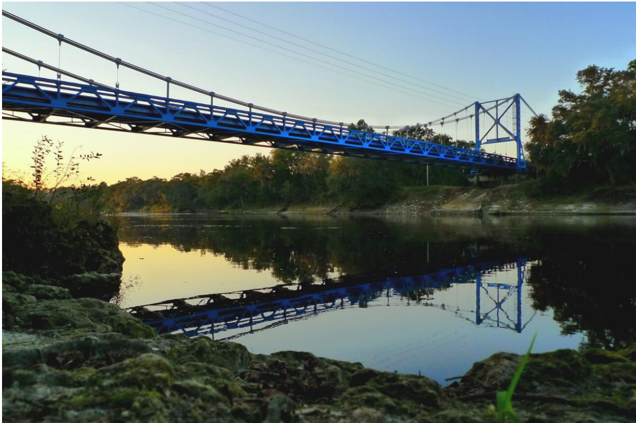
Hal W. Adams Bridge, State Road 51 over Suwannee River
