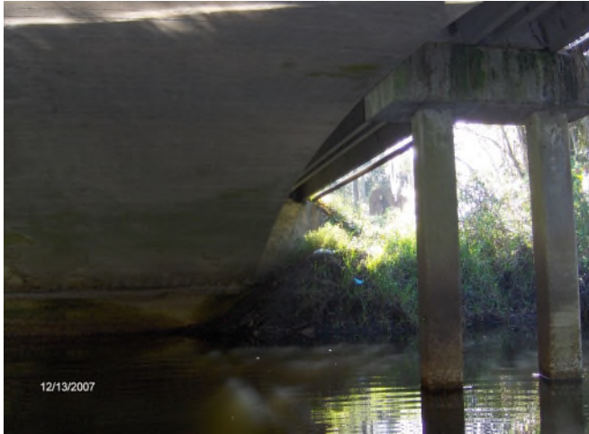
Figure 4 – Arch widened from below
