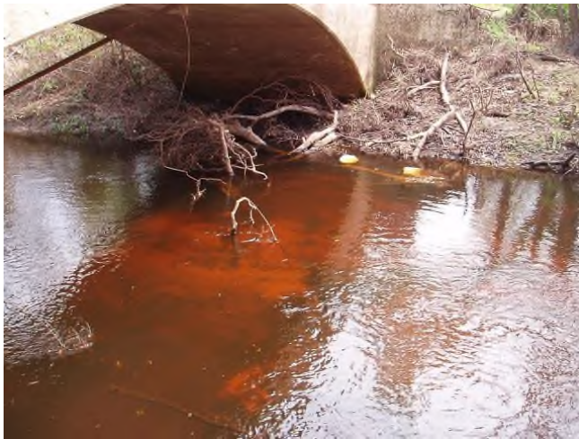
Figure 1 – Arch no cantilever
