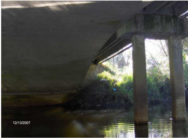
Figure 4 – Arch widened from below
